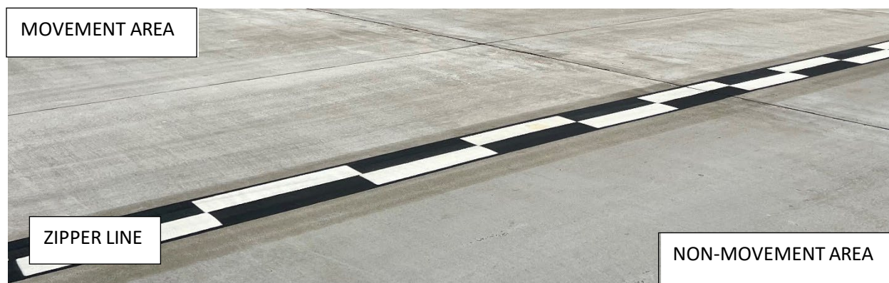
Figure 5 – Dashed Taxiway Edge Markings and Black/White Zipper Marking
