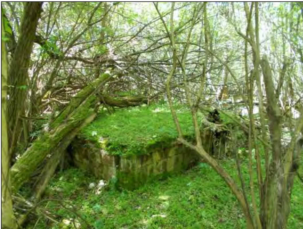
Figure 5-15. Flagstone veneer on south portion of the foundation, view northwest (DSCN2592).
