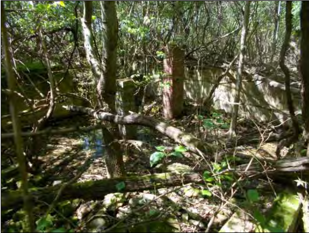
Figure 5-13. Locus 4 foundation and free standing chimney, view southwest (DSCN2594).
