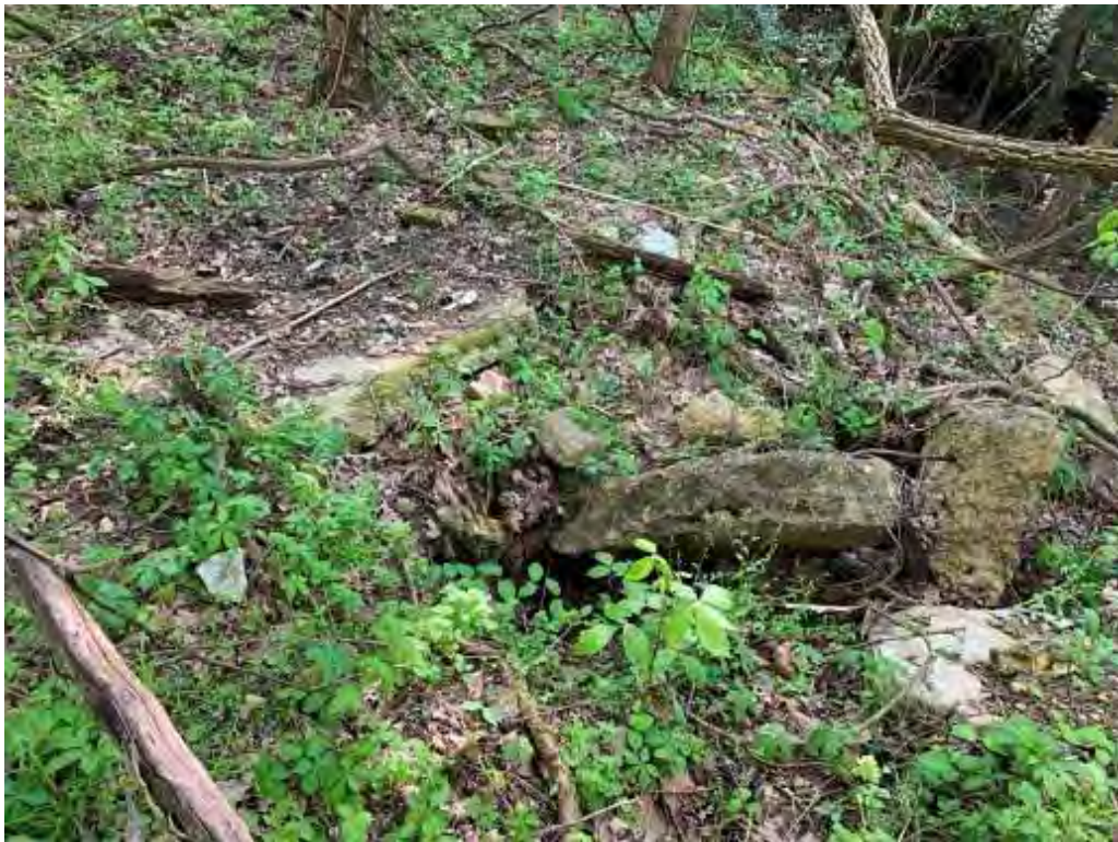
Photo 2: View of the broken concrete presumed to be from a former building structure in the north-central portion of the subject property.
