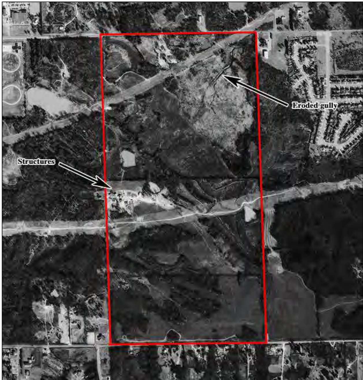
Figure 4-12. A portion of the 1990 air photo with the MSCAA Holmes Road tract highlighted.
