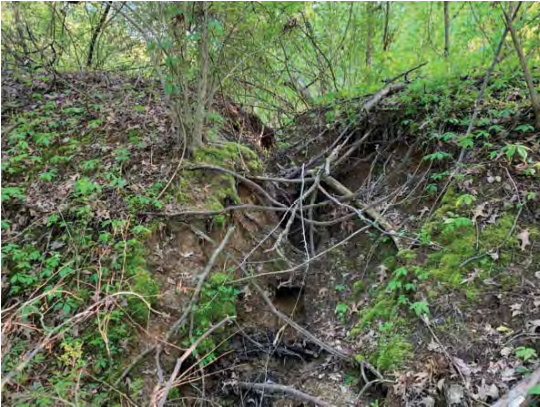
Photo 9: View of breach in Pond 3 berm, which drains into WWC 7, facing south. (34.99942°, -89.969566°)
