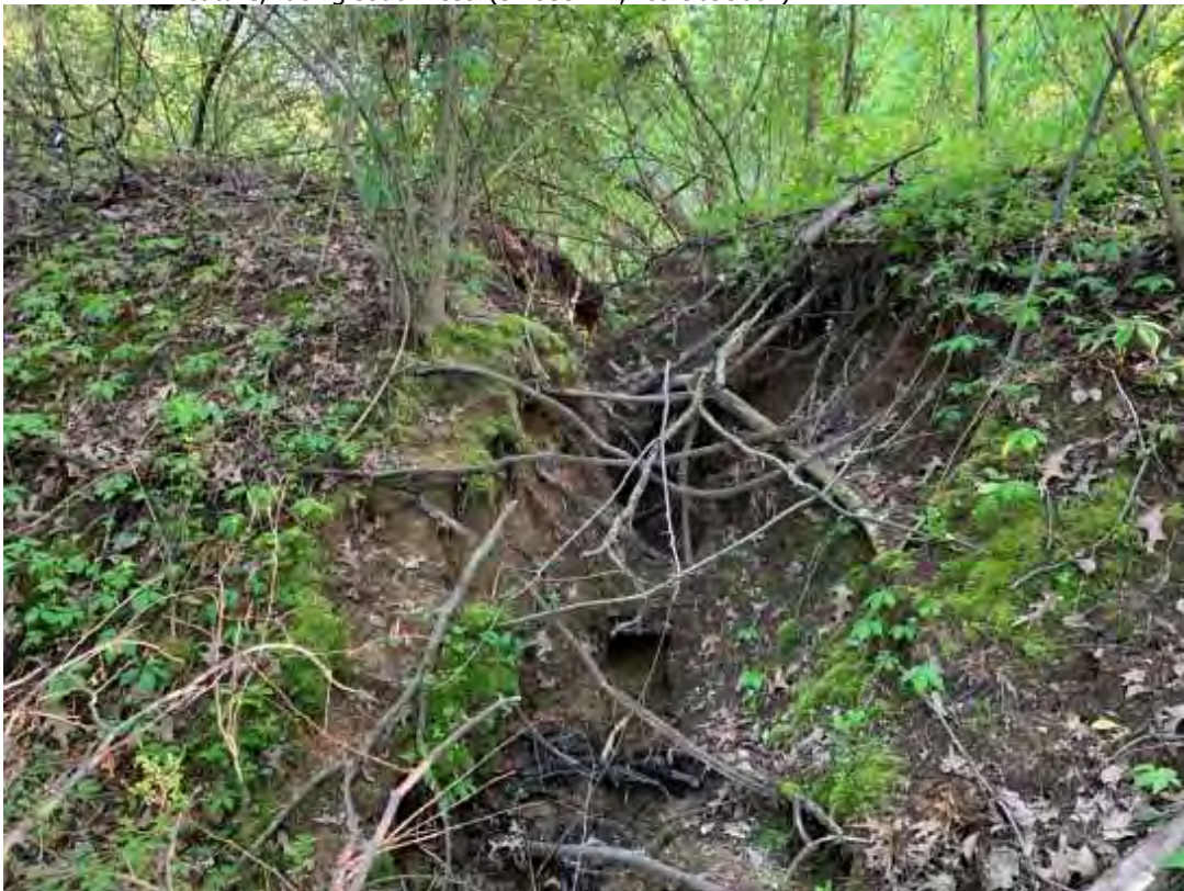
Photo 10: View of breach in Pond 3 berm, which drains into a non-WOTUS linear drainage feature, facing south toward the pond. (34.99942°, -89.969566°)
