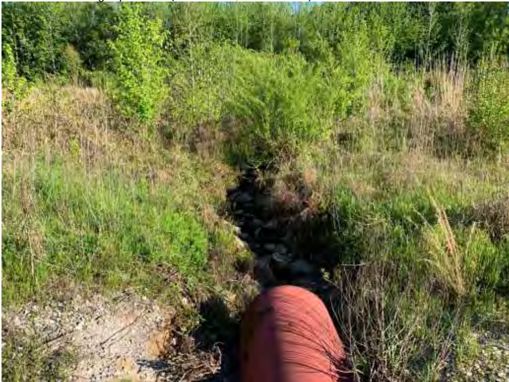
Photo 33: View of Stream 1 historical impact, where it enters an approximately 200-foot-long culvert at the south utility line easement, facing south. (34.997768°, -89.96608°)
