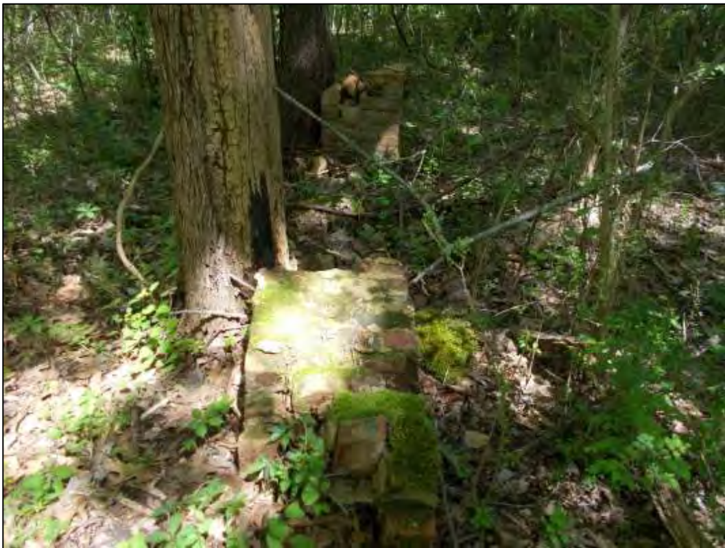
Figure 5-08. Chimney fall at Locus 2, view north (DSCN2572).
