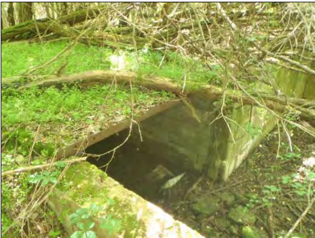
Figure 5-14. Locus 4 southeast corner of foundation, view southwest (P409641).
