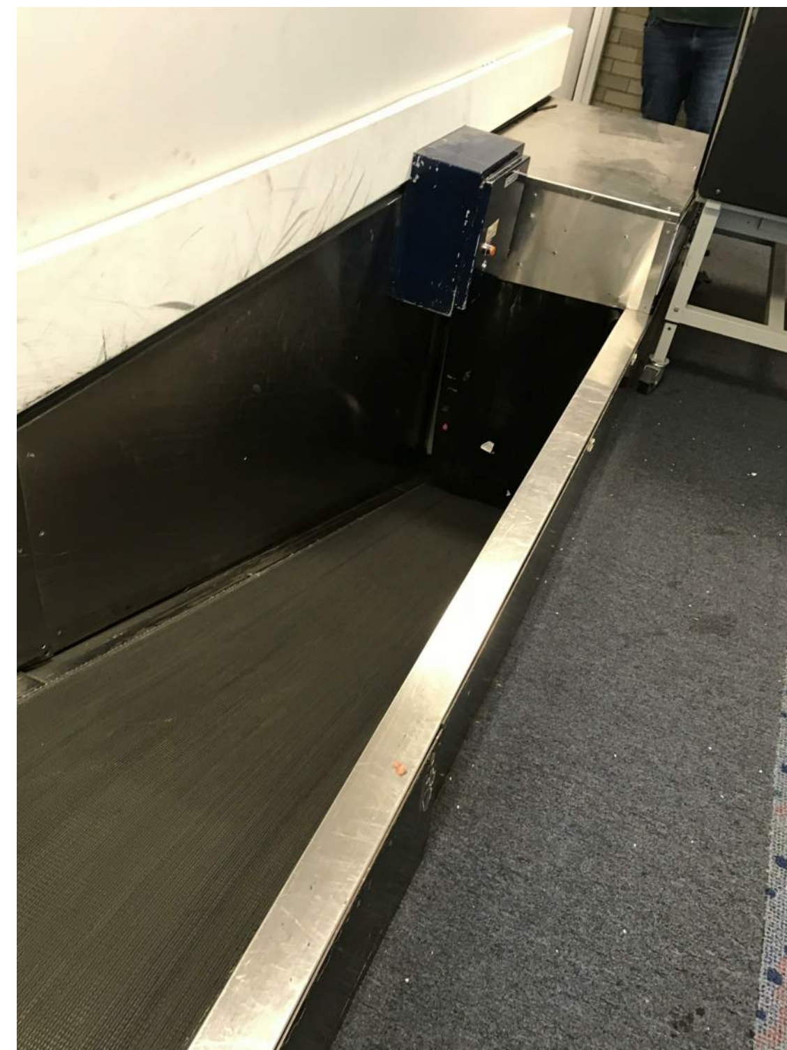
PICTURE 5 THE SCOPE OF WORK FOR DESIGN BUILD CONTRACTOR SHALL INCLUDE THE REPLACEMENT OF THE SECURITY ROLLUP GATE AS WELL AS THE INCLINED BELT AS PART OF THE BELT REPLACEMENT PACKAGE AT THE CONCOURSE LEVEL. THE NEW GATE SHALL BE HEAVY INDUSTRIAL DUTY, FIRE AND SECURITY ELECTRICAL ROLL UP DOOR WITH INTEGRATED CONTROL WITH THE BELT SYSTEM. CONTRACTOR ALSO TO PROVIDE AND INSTALL OSHA COMPLIANT GUARD/BARRIER AT INCLINED BELT FOR FALL PROTECTION.
