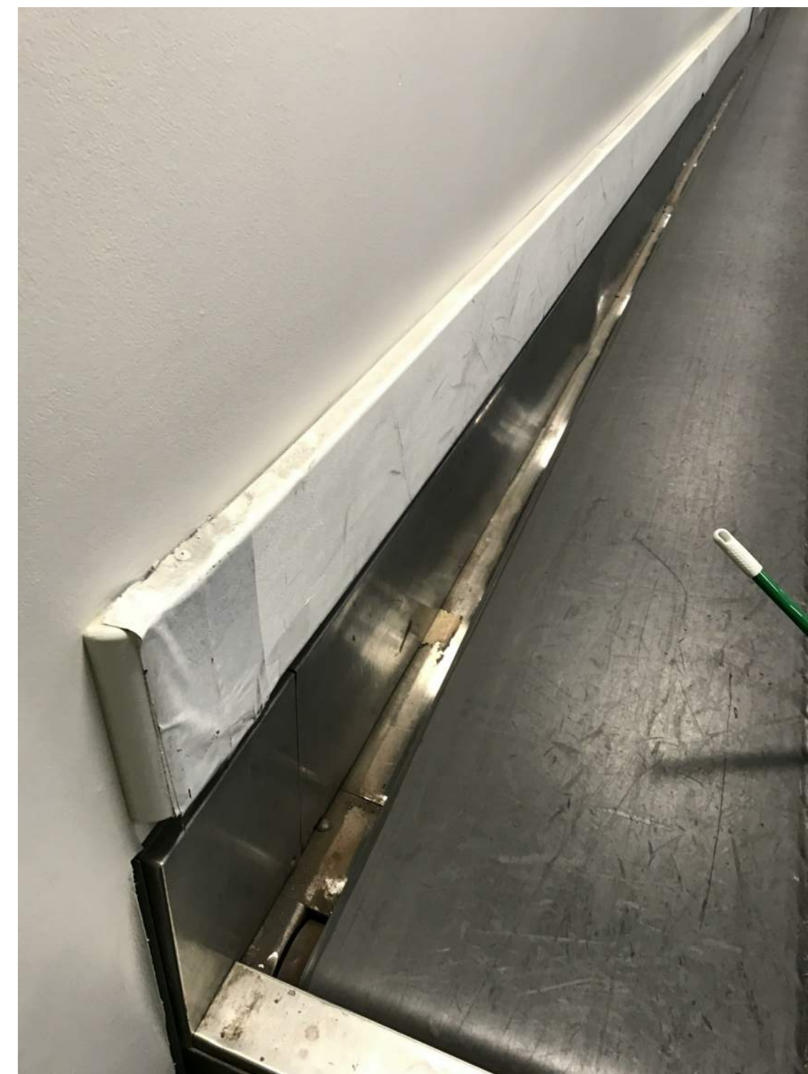
PICTURE 2 REMOVE AND REPLACE THE ENTIRE BELT SYSTEM AND ALL ASSOCIATED TRIMS. THE SCOPE OF WORK SHALL INCLUDE REPAINTING OF THE ENTIRE WALL BEHIND THE NEW REPLACEMENT.
