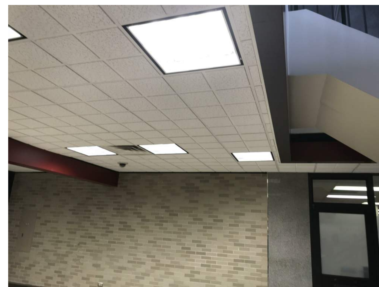
TIE IN NEW CEILING GRID SYSTEM IN THE NEWLY RESTORED SPACE TO MATCH EXISTING 2X4 GRID SYSTEM, TILE TYPE AND ORIENTATION. THE NEW LIGHT FIXTURES SHALL MATCH THE EXISTING 2X2 FIXTURES WITH THE 9 GRID PARABOLIC LENS.
