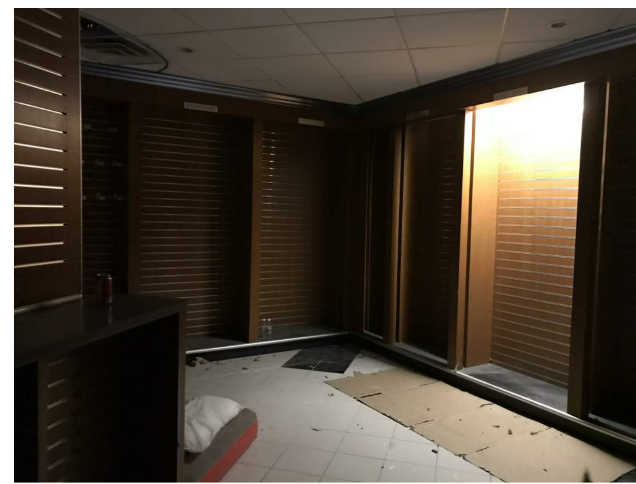
REMOVE ALL EXISTING SHELVING AND DISPLAY MILLWORK. REMOVE FLOOR AND CEILING TILE SYSTEM.
