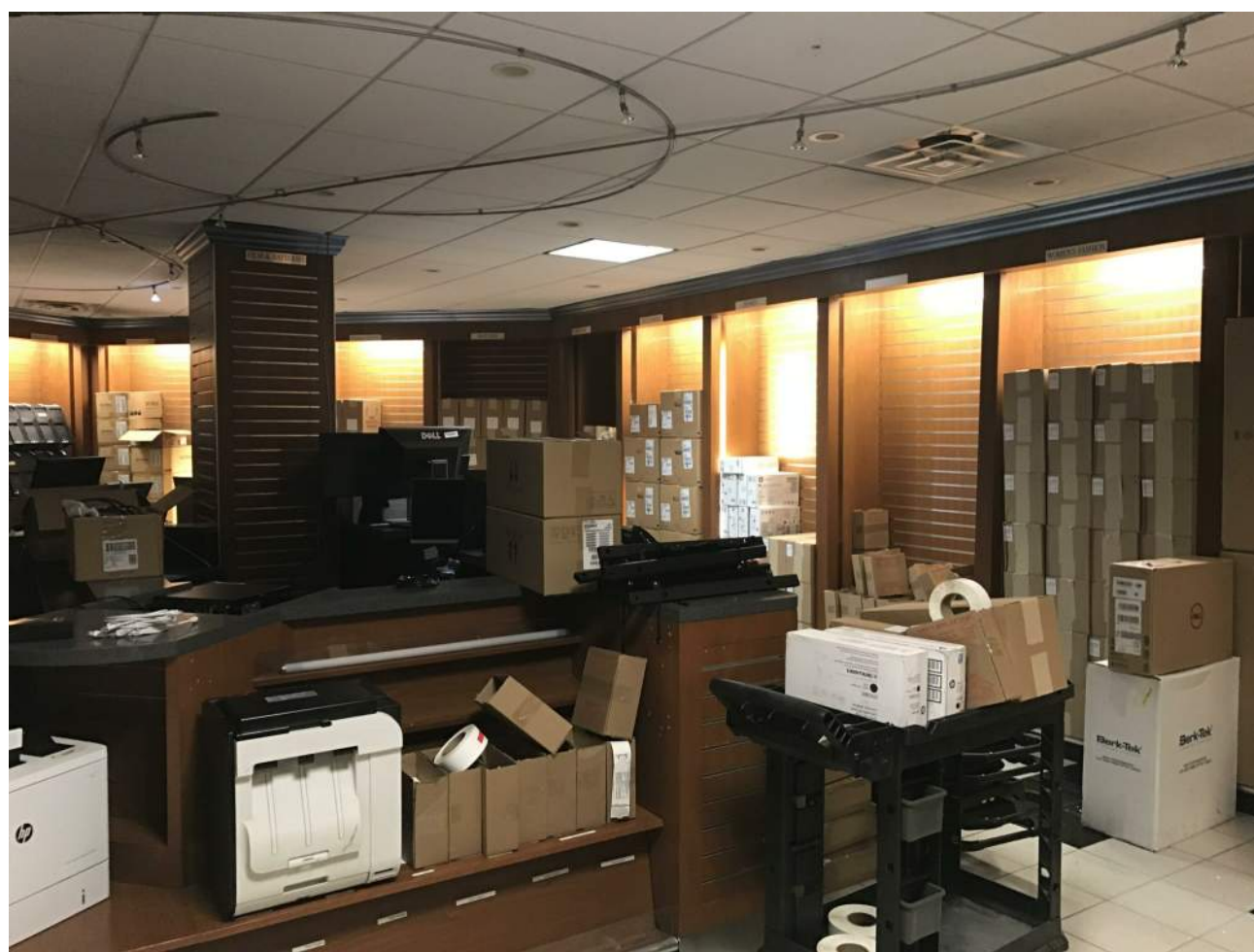
REMOVE ALL EXISTING SHELVING AND DISPLAY MILLWORK. REMOVE FLOOR AND CEILING TILE SYSTEM.
