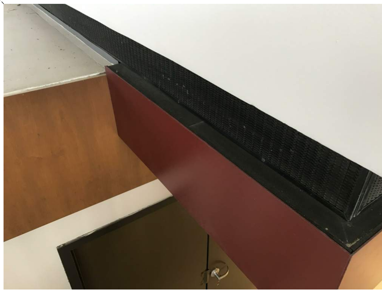
CLOSE UP VIEW OF THE COLOR BAND. INSTALL NEW COLOR BANDING AT THE BOTTOM OF THE MEZZANINE TO MATCH EXISTING ADJACENT.
