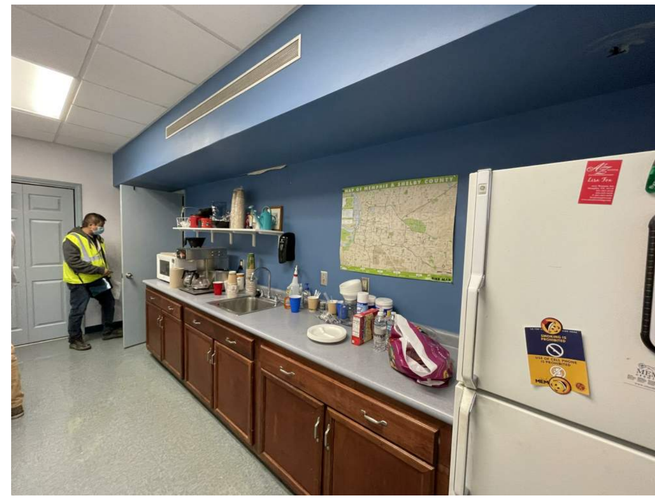
EXISTING MILLWORK TO BE REMOVED. REMOVE FLOOR FINISHES AND RESTORE THE ORIGINAL TERRAZZO FLOOR SYSTEM. SPOT REPAIR AS NEEDED.
