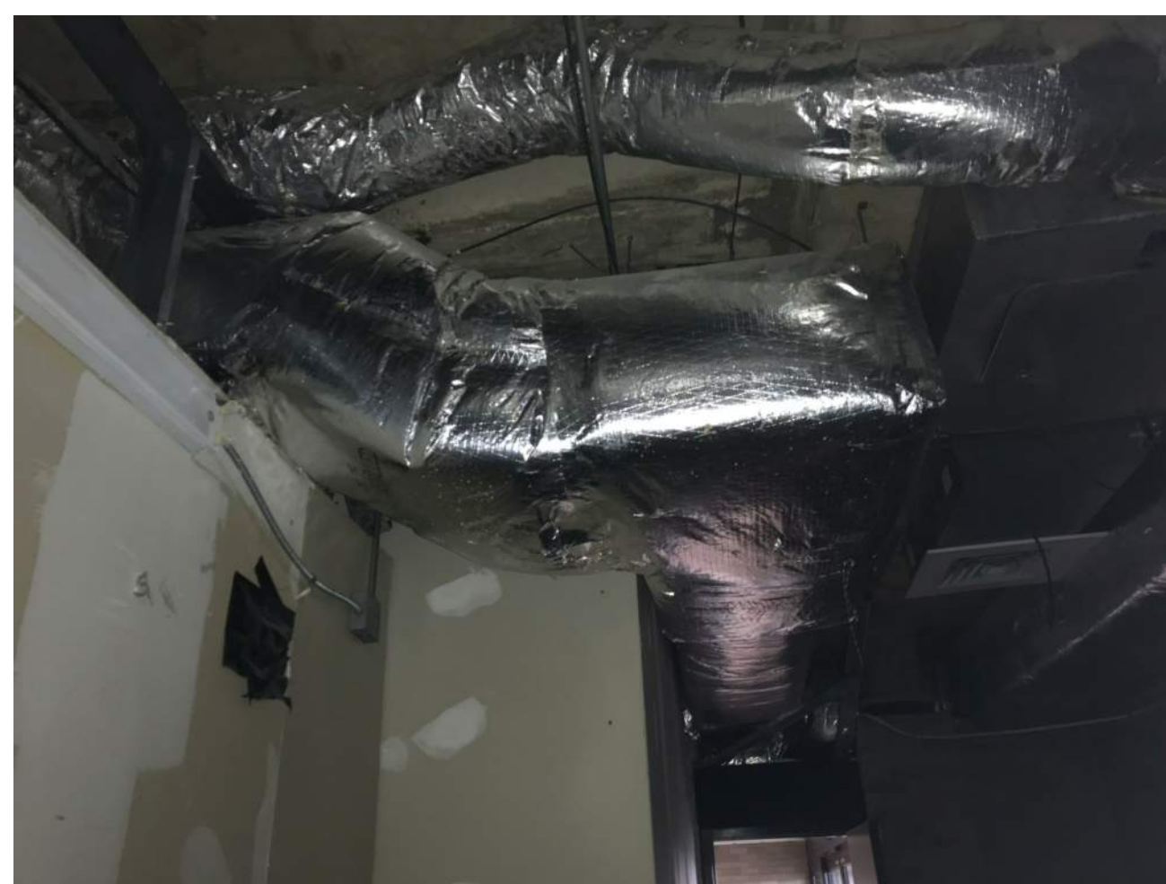
REROUTE THE EXISTING DUCT WORK AND VAV BOX HOT WATER LINE AS NEEDED IN THE STORAGE ROOM BEHIND TO PROVIDE VERTICAL CLEARANCE FOR THE APPROXIMATE 9'-0" LAY IN CEILING HEIGHT TO MATCH ALL EXISTING ADJACENT CEILING.
