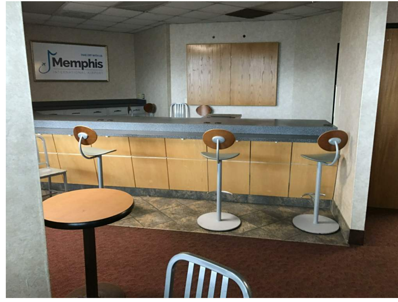
EXISTING MILLWORK TO BE REMOVED. REMOVE FLOOR FINISHES AND RESTORE THE ORIGINAL TERRAZZO FLOOR SYSTEM. SPOT REPAIR AS NEEDED.
