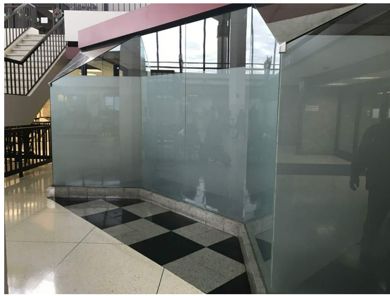
EXISTING GLASS PARTITION WALL AND BOTTOM CURBS TO BE REMOVED. REMOVE FLOOR TILES AND RESTORE THE ORIGINAL TERRAZZO FLOOR SYSTEM. SPOT REPAIR AS NEEDED.
