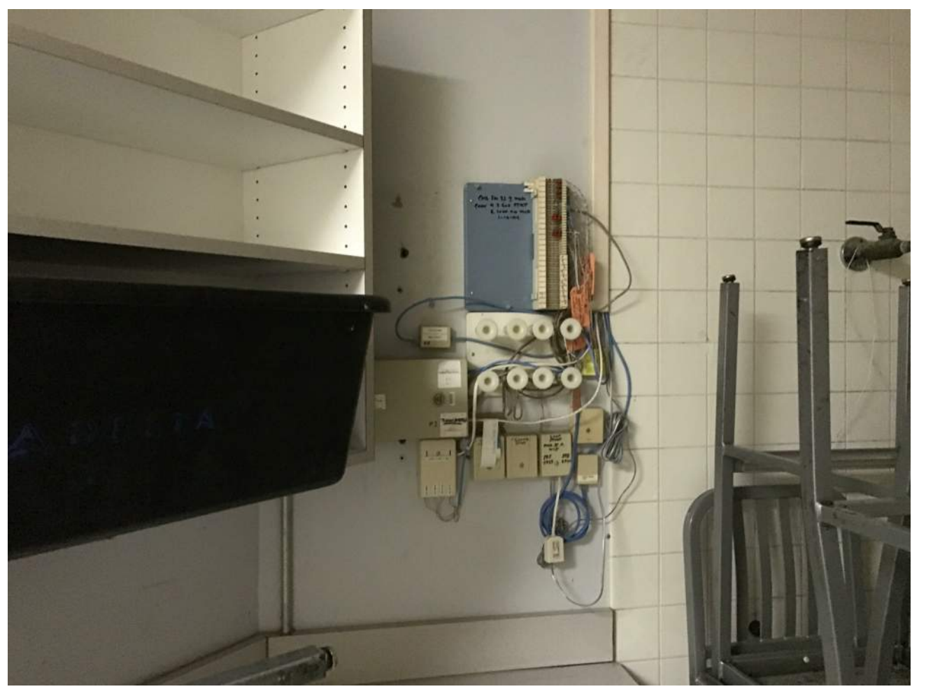
REMOVE ABANDONED NETWORK WIRING. CONFIRM WITH AIRPORT MAINTENANCE BEFORE REMOVAL. CAP OFF THE UTILITY CONNECTION FOR ORIGINAL APPLIANCE.
