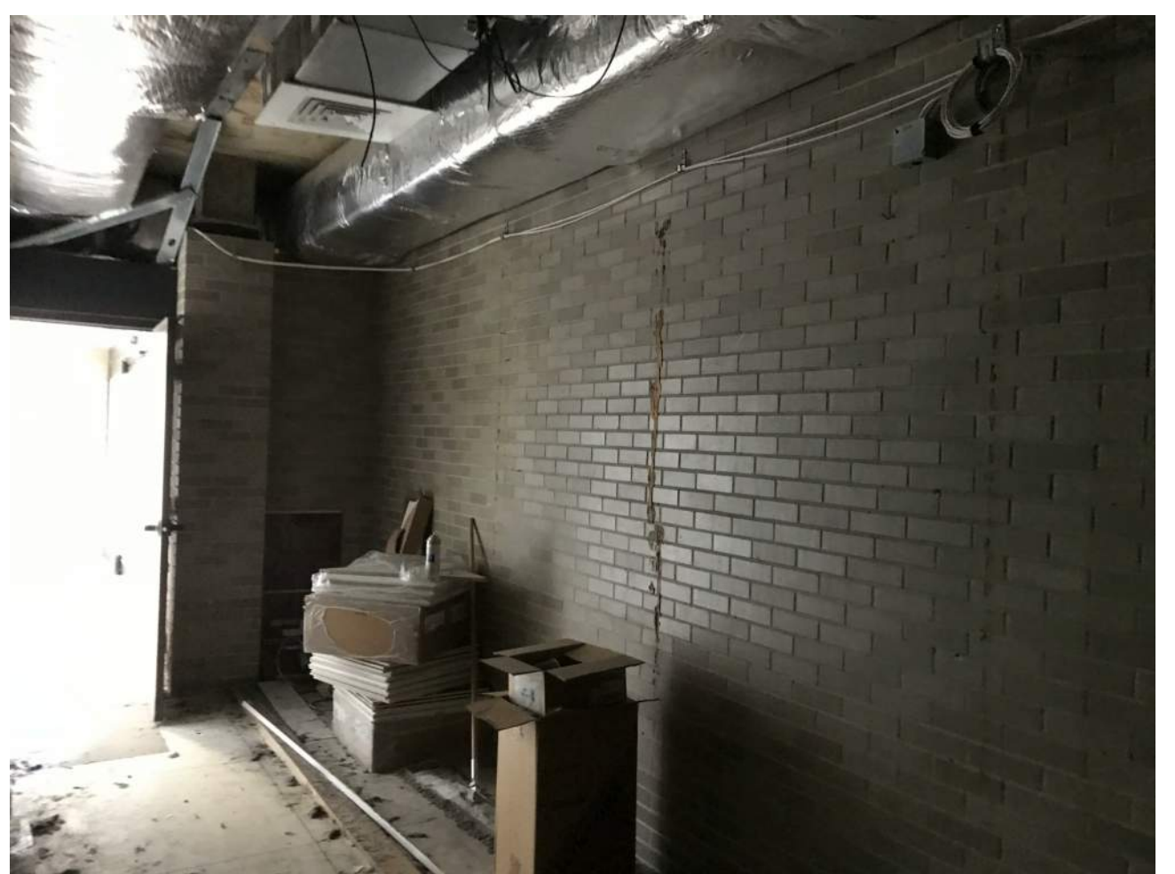
SPOT REPAIR EXISTING BRICK VENEER FINISH AFTER REMOVAL OF INTERIOR FINISHES. THE AIRPORT AUTHORITY SHALL PROVIDE THE BRICK MASONRY UNITS NEEDED FOR THE REPAIR.
