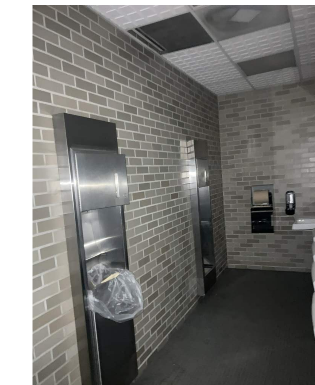
PICTURE B EXISTING CONDITION OF THE MENS RESTROOM AT TERMINAL C FOR ALTERNATE ONE. THE RESTROOM HAS NOT BEEN IN USE.
