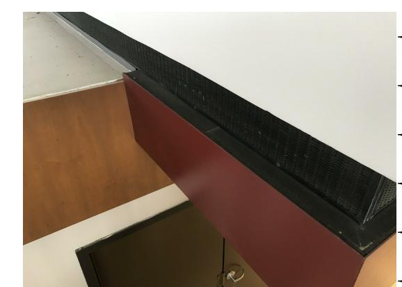
PROTECT THE VENTILATION BAND GRILLE DURING CONSTRUCTION TO PREVENT MIGRATION OF CONSTRUCTION DUST INTO THE AIR HANDLING SYSTEM
