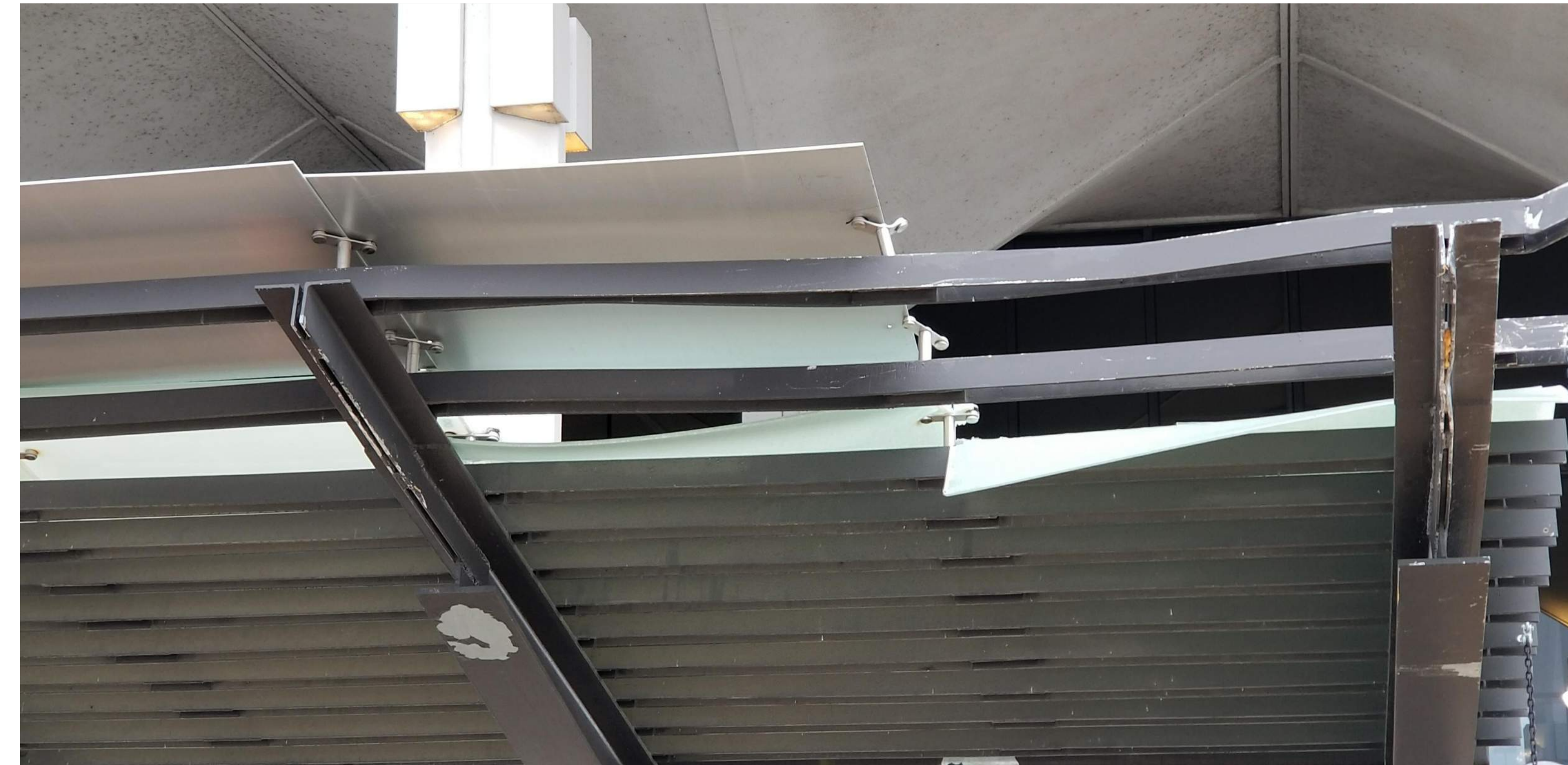
FIELD VERIFY THE EXACT EXTENT OF THE ACTUAL DAMAGE AND REPAIR NEEDED TO ENSURE PROPER FITMENT AND SATISFACTORY OVERALL DAMAGE REPAIR. TOUCH UP OR REPAINT THE STEEL MEMBERS TO MATCH EXISTING ADJACENT FINISH
