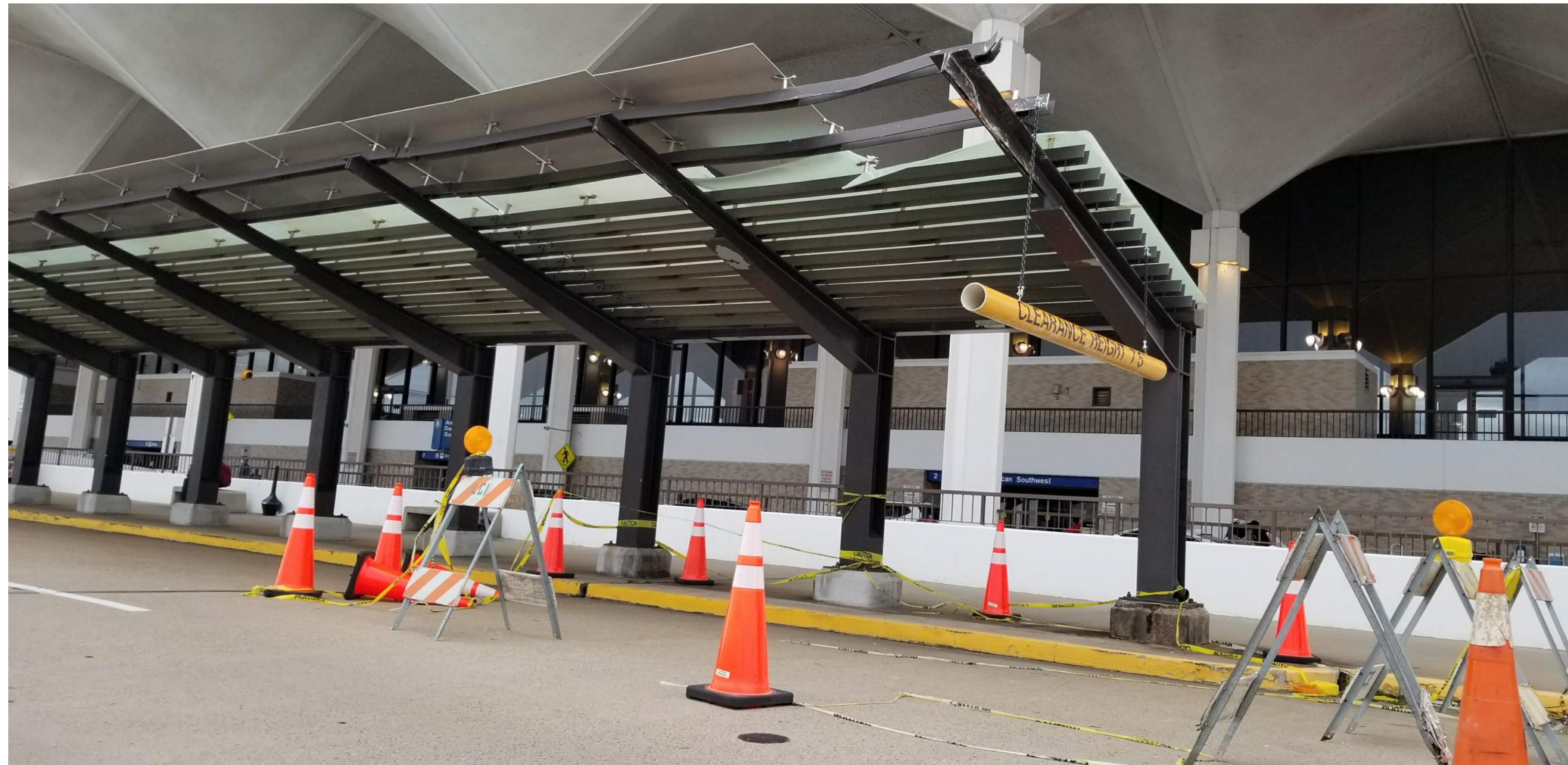
THE DAMAGE IS MAINLY LIMITED TO THE FRONT APPROACHING CORNER AND THE CONNECTED SECONDARY MEMBERS. COORDINATE WITH AIRPORT FOR THE EXACT LIMIT OF THE WORK ZONE TO MINIMIZE DISRUPTION TO THE VEHICULAR TRAFFIC FLOW
