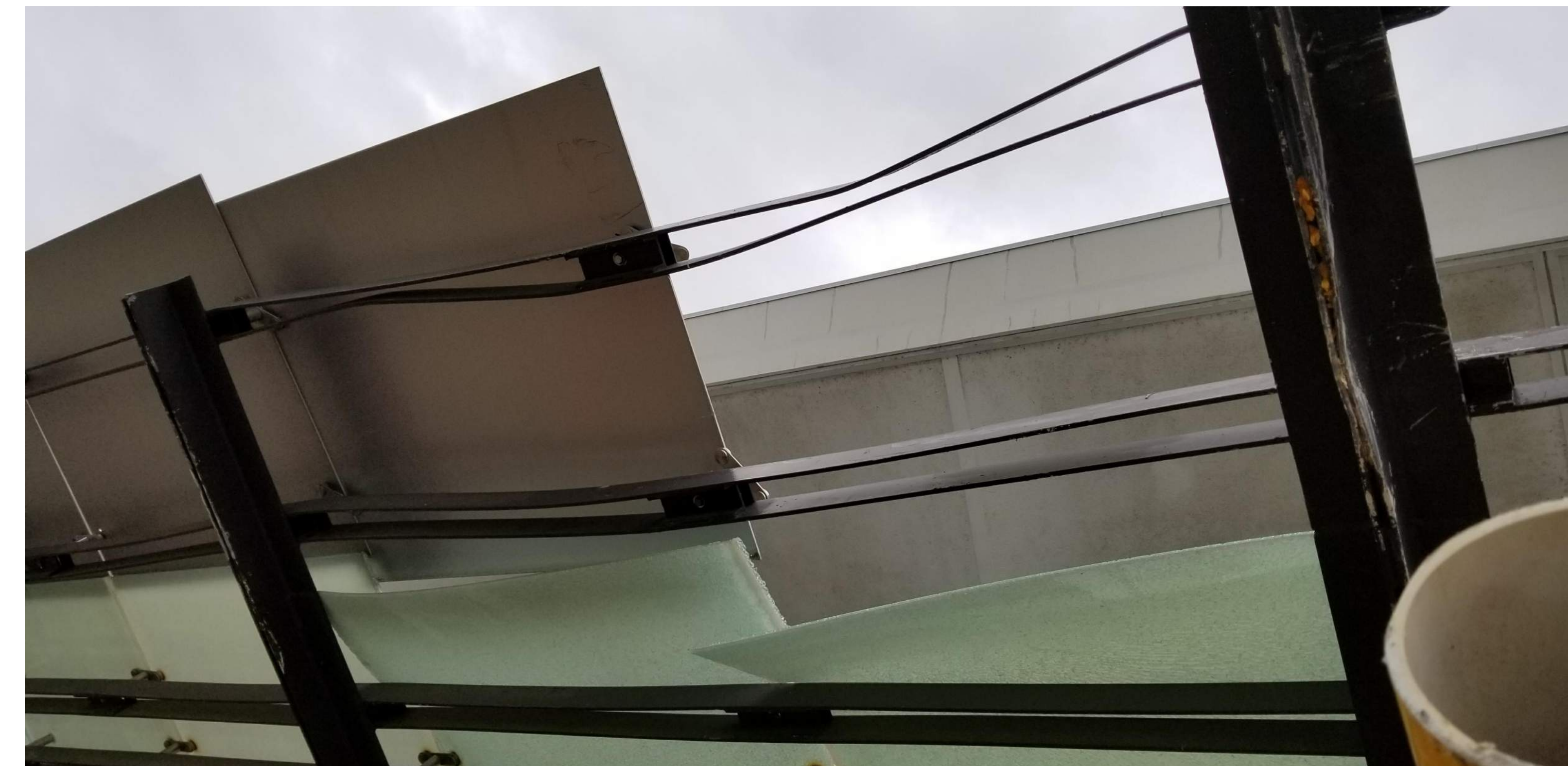
REMOVE DAMAGED STEEL SUPPORT MEMBERS UP TO THE FIRST EXPANSION JOINT. REPLACE WITH EXACT SAME MEMBER. SEE A1.2 AND A1.3 FOR RECORD OF STRUCTURAL AND ARCHITECTURAL DESIGN BY THE ORIGINAL DESIGNER.
