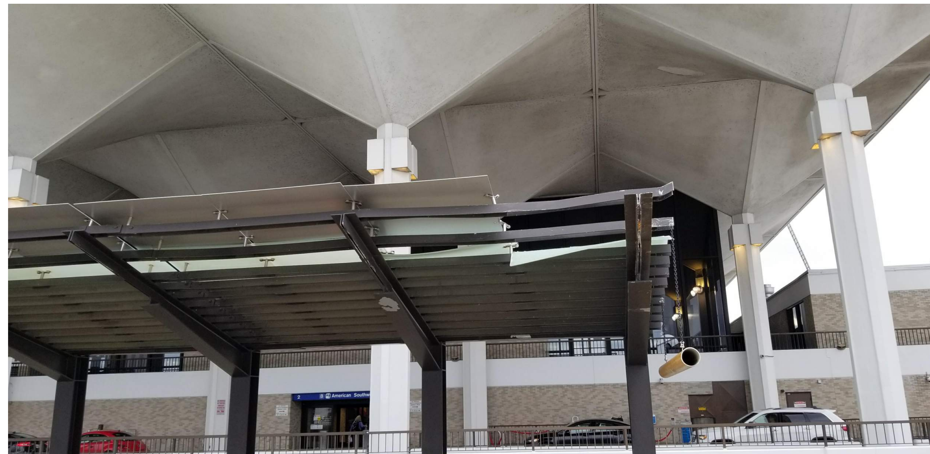
DAMAGED LAMINATED GLASS AND ANY LOOSE FASTENERS OR SHARP METAL SCRAPS SHALL BE REMOVED CAREFULLY SO AS NOT TO SCATTER OVER THE VEHICULAR PATH THAT MAY CAUSE TIRE DAMAGE TO PASSING TRAFFIC.
