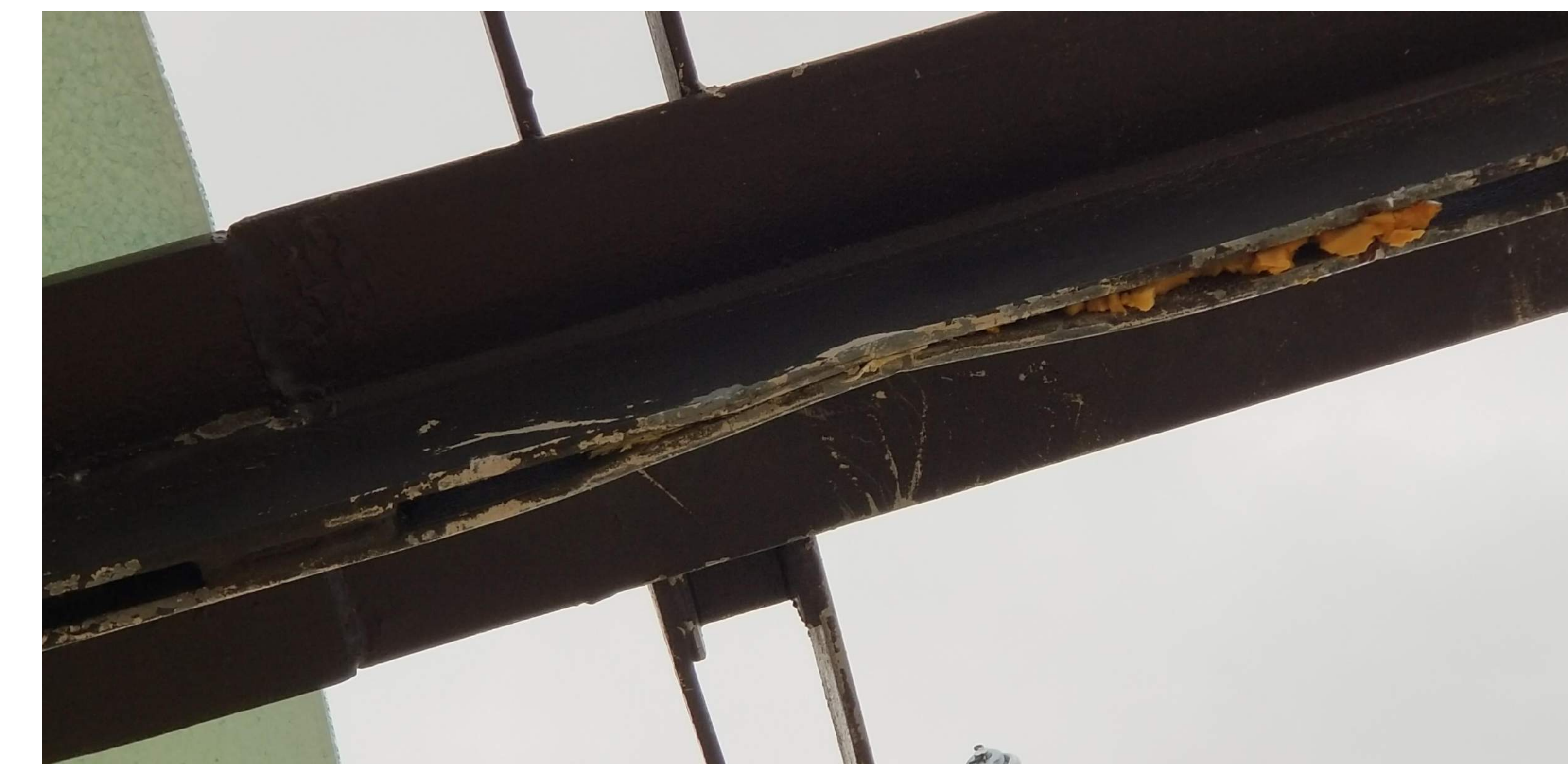
REPAIR STEEL SUPPORT EXTENSIONS WHEREVER FEASIBLE. IF REPAIR IS NOT POSSIBLE, CUT AND REPLACE WITH THE SAME ORIGINAL DESIGN. PROTECT THE PEDESTRIAN AND TRAFFIC WHEN CUTTING OR GRINDING IS NECESSARY. COORDINATE WITH AIRPORT FOR APPROVAL WHEN WELDING IS NECESSARY TO AVOID PEDESTRIAN EXPOSURE OF BRIGHT LIGHT FROM WELDING ACTIVITIES.
