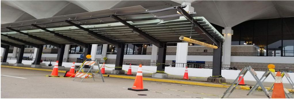
THE DAMAGE IS MAINLY LIMITED TO THE FRONT APPROACHING CORNER AND THE CONNECTED SECONDARY MEMBERS. COORDINATE WITH AIRPORT FOR THE EXACT LIMIT OF THE WORK ZONE TO MINIMIZE DISRUPTION TO THE VEHICULAR TRAFFIC FLOW.
