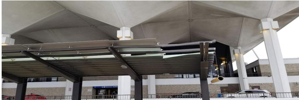
DAMAGED LAMINATED GLASS AND ANY LOOSE FASTENERS OR SHARP METAL SCRAPS SHALL BE REMOVED CAREFULLY SO AS NOT TO SCATTER OVER THE VEHICULAR PATH THAT MAY CAUSE TIRE DAMAGE TO PASSING TRAFFIC.
