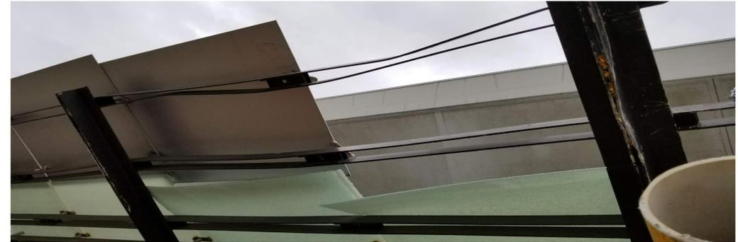
REMOVE DAMAGED STEEL SUPPORT MEMBERS UP TO THE FIRST EXPANSION JOINT. REPLACE WITH EXACT SAME MEMBER. SEE A1.2 AND A1.3 FOR RECORD OF STRUCTURAL AND ARCHITECTURAL DESIGN BY THE ORIGINAL DESIGNER.
