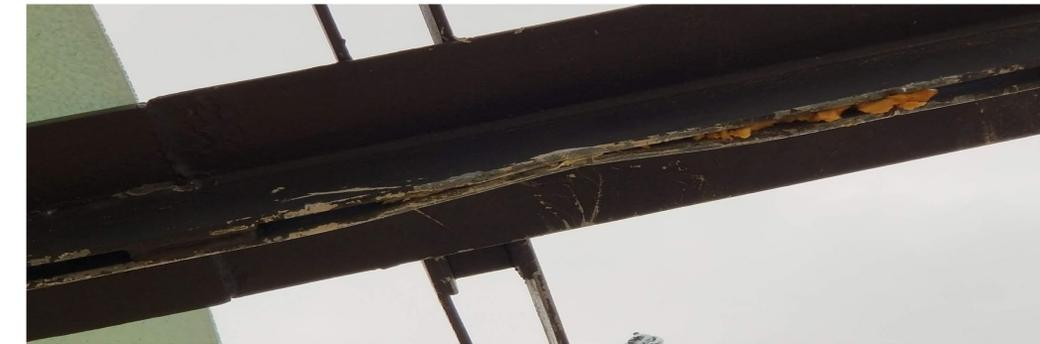
REPAIR STEEL SUPPORT EXTENSIONS WHEREVER FEASIBLE. IF REPAIR IS NOT POSSIBLE, CUT AND REPLACE WITH THE SAME ORIGINAL DESIGN. PROTECT THE PEDESTRIAN AND TRAFFIC WHEN CUTTING OR GRINDING IS NECESSARY. COORDINATE WITH AIRPORT FOR APPROVAL WHEN WELDING IS NECESSARY TO AVOID PEDESTRIAN EXPOSURE OF BRIGHT LIGHT FROM WELDING ACTIVITIES.
