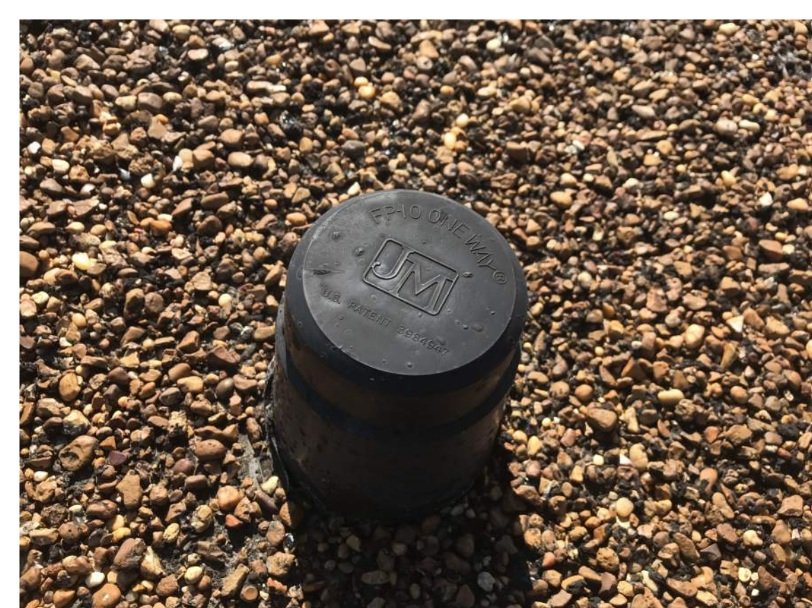
PHOTO 3 EXISTING ROOF RELIEF VENTS SHALL BE REMAIN. REPLACE ONLY AS NEEDED
