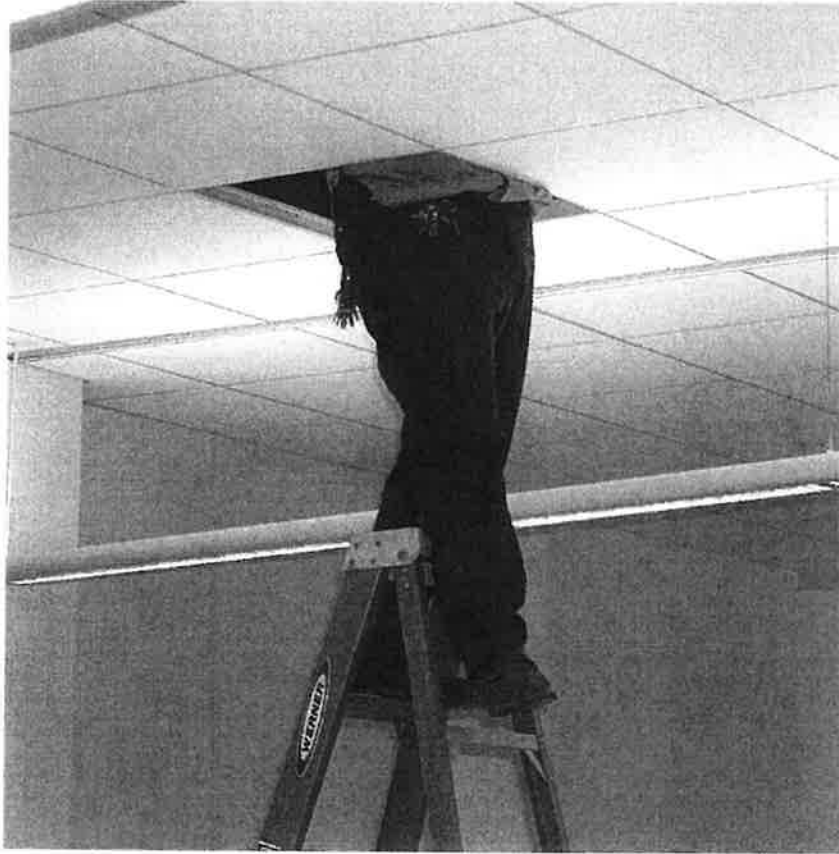
Figure 8 Example of what not to do. Never stand on the top two steps of a step ladder
