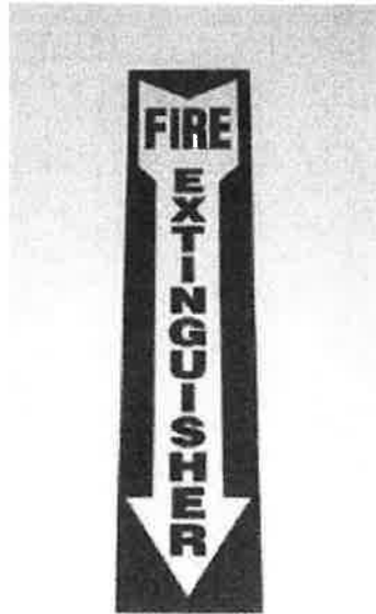
Figure 11 Sign above a fire extinguisher
