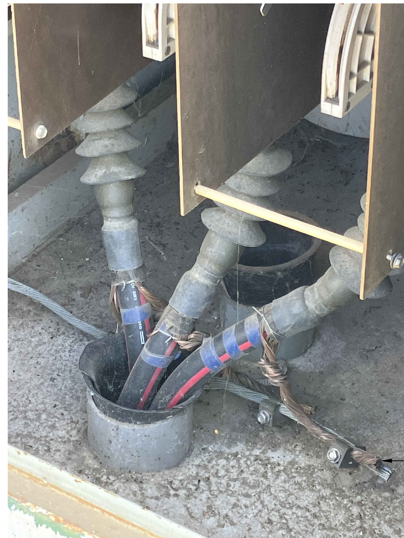
2 EXISTING INCOMING CONDUCTORS SCALE: NONE
