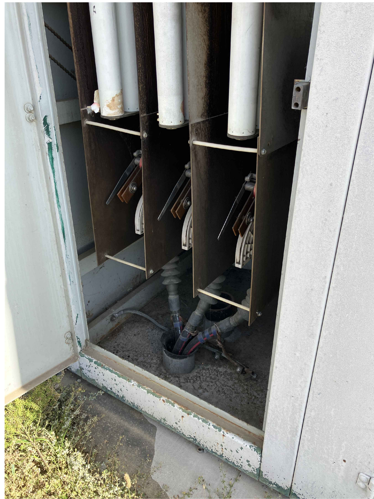
1 EXISTING MAIN CAPACITOR BANK SWITCH SCALE: NONE
