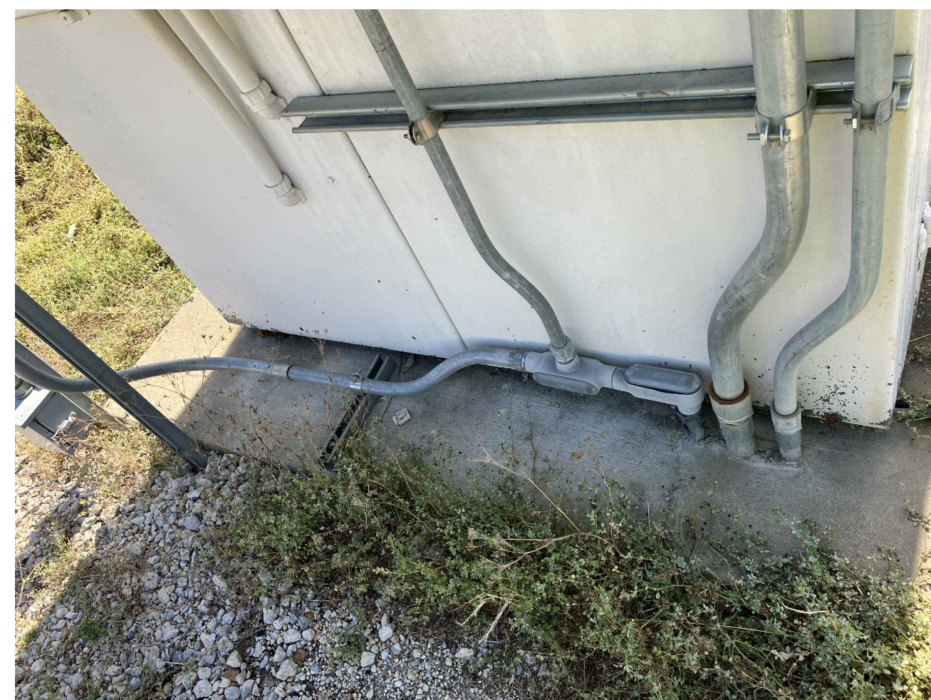
4 EXISTING CONTROLS CONDUITS SCALE: NONE
