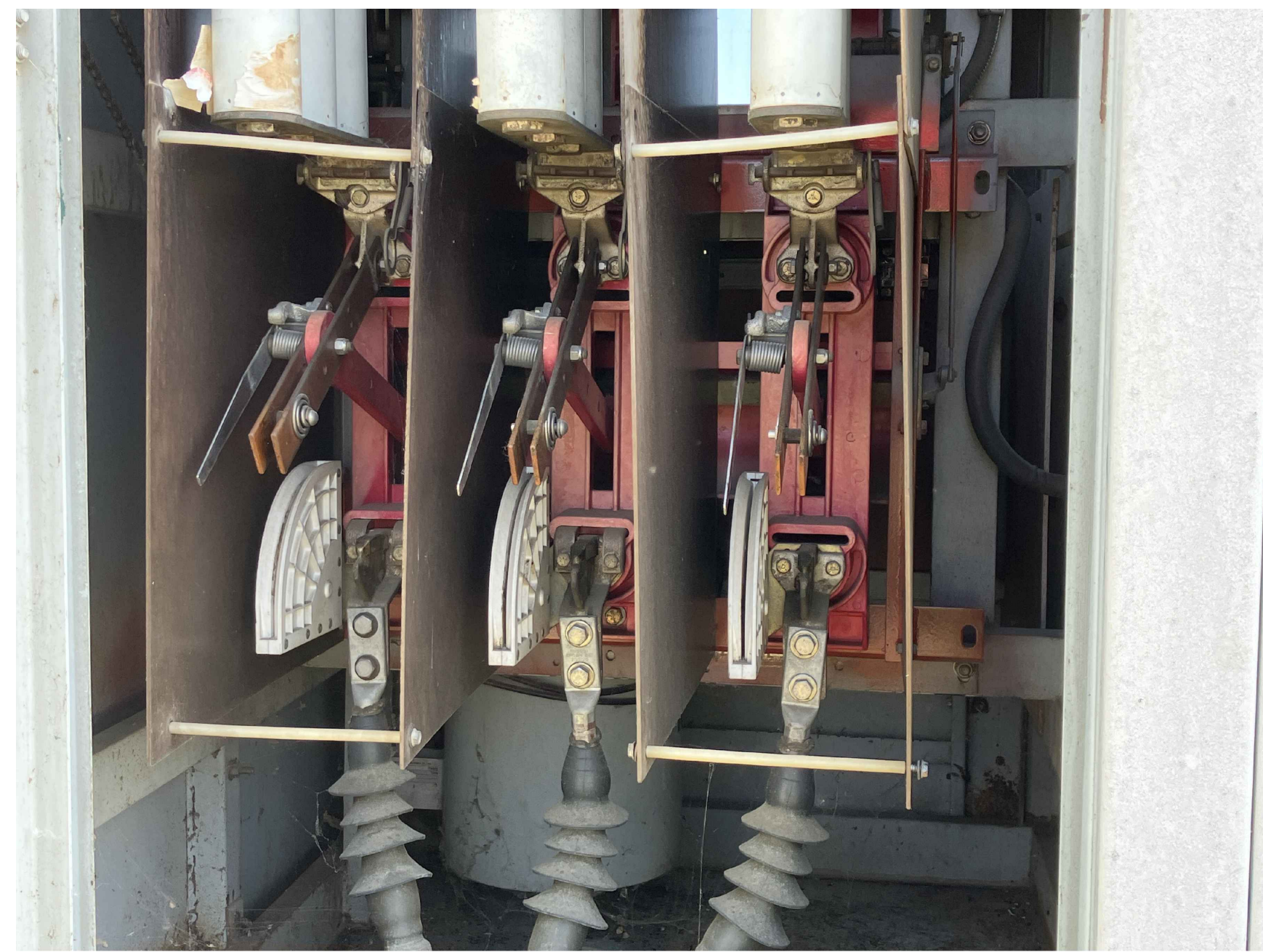
4 EXISTING MAIN CAPACITOR BANK SWITCH SCALE: NONE
