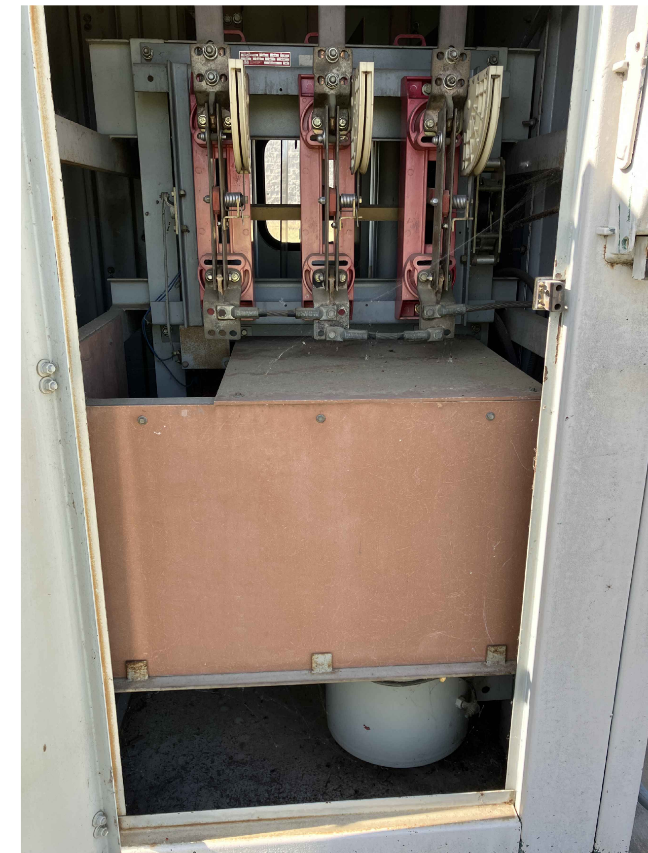
5 EXISTING GROUNDING SWITCH SCALE: NONE
