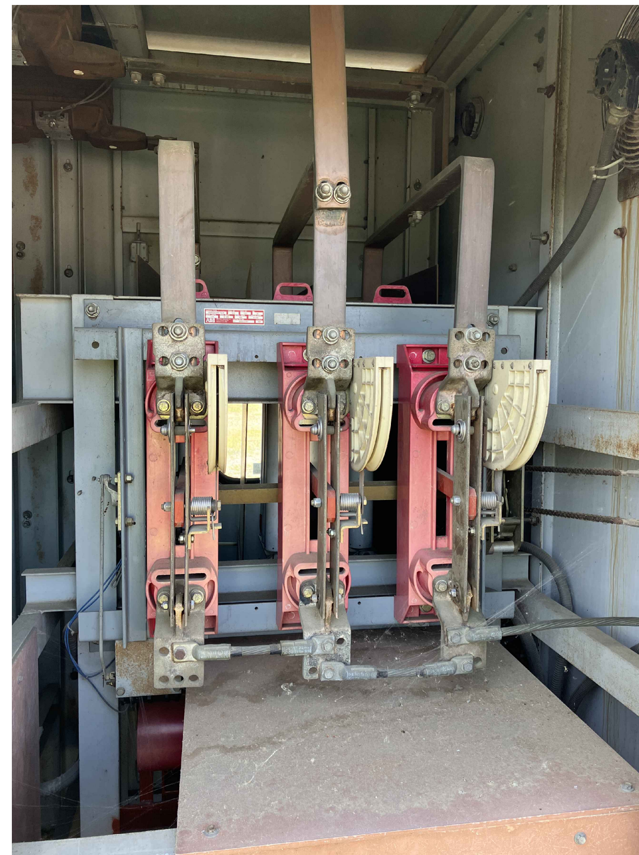
4 EXISTING GROUNDING SWITCH SCALE: NONE
