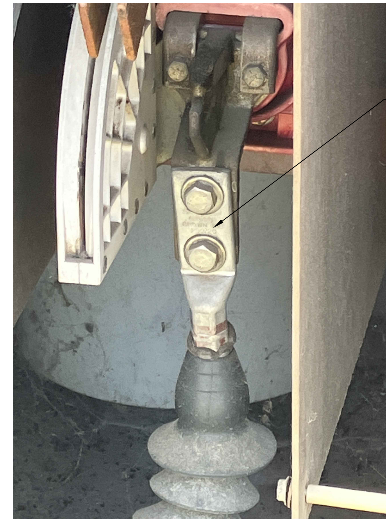
6 EXISTING CAPACITOR BANK BOLTED TERMINAL CONNECTION SCALE: NONE
