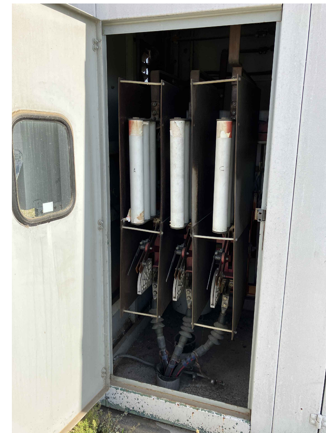
3 EXISTING MAIN CAPACITOR BANK SWITCH SCALE: NONE
