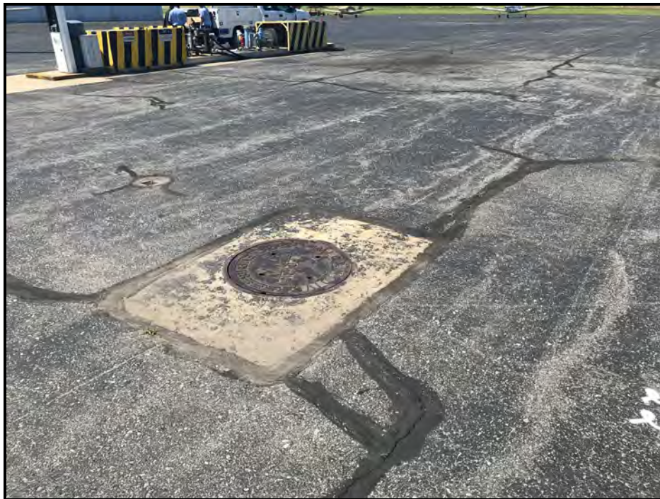
Photo 4 – APME-001 Looking SW Towards Fueling Area
