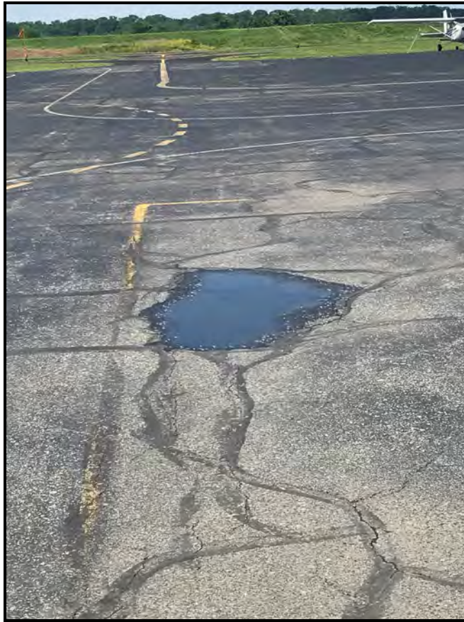
Photo 3 APME-001 Looking W
