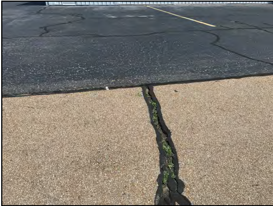
Photo 8 Interface of APME-001 and APME-002 Looking S
