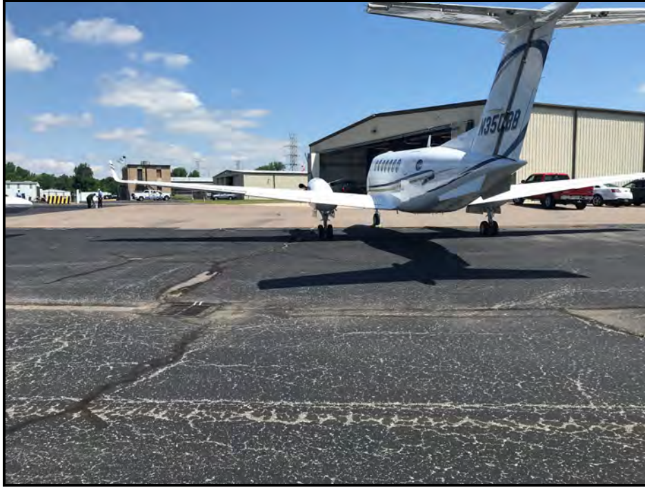
Photo 7 - APME-001 Looking N to APME-002
