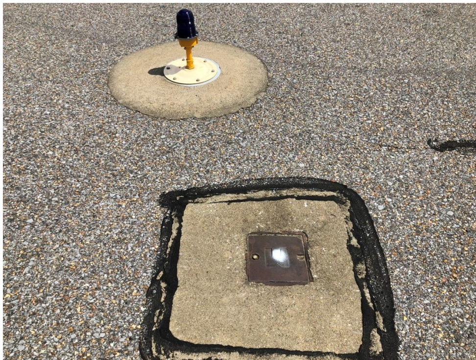
Existing underdrain cleanout (typical)
