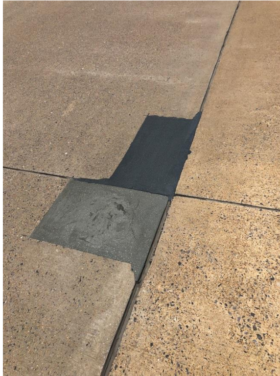
Delpatch corner break/spall repair
