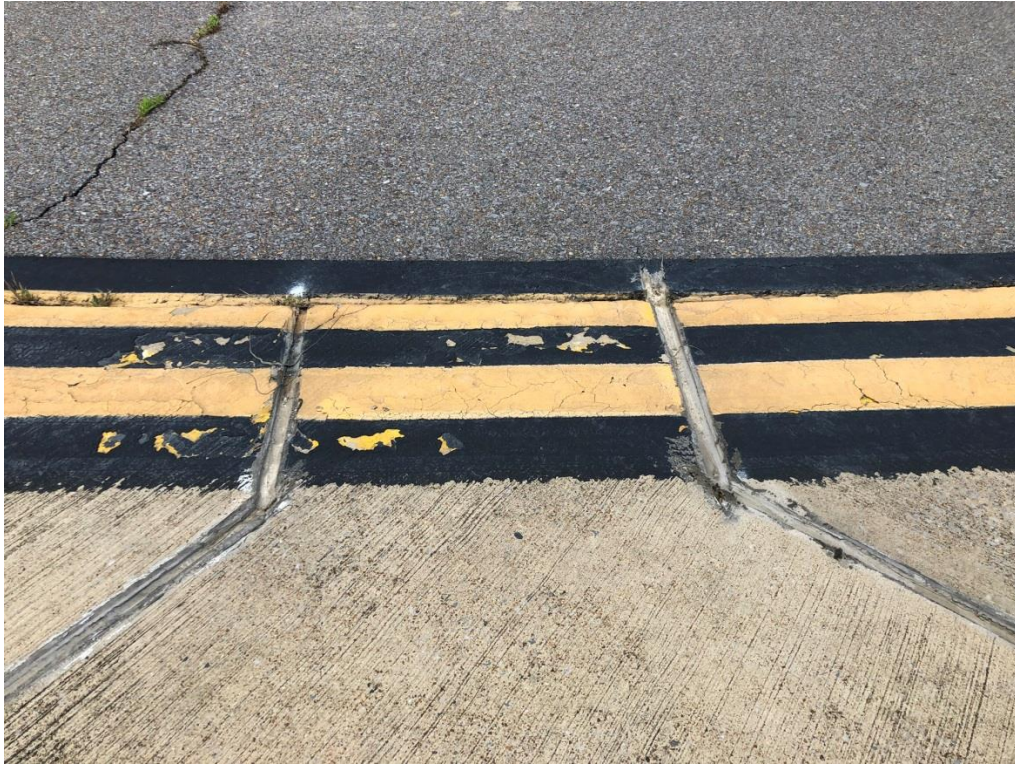
Typical slab joint transition
