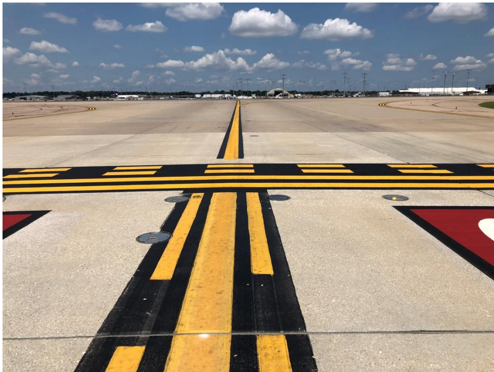
In-pavement Runway Guard Lights @ 9-27 Hold
