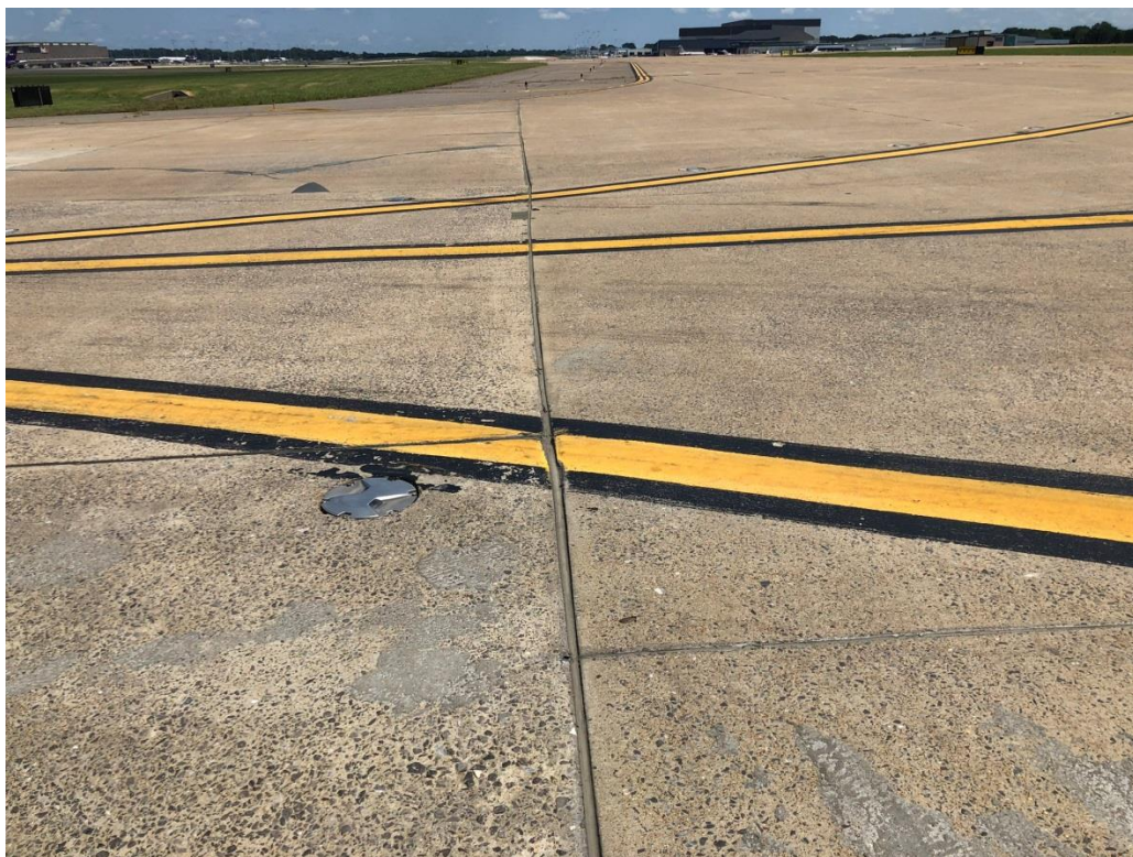
Thickened-edge expansion joint along Taxiway Alpha
