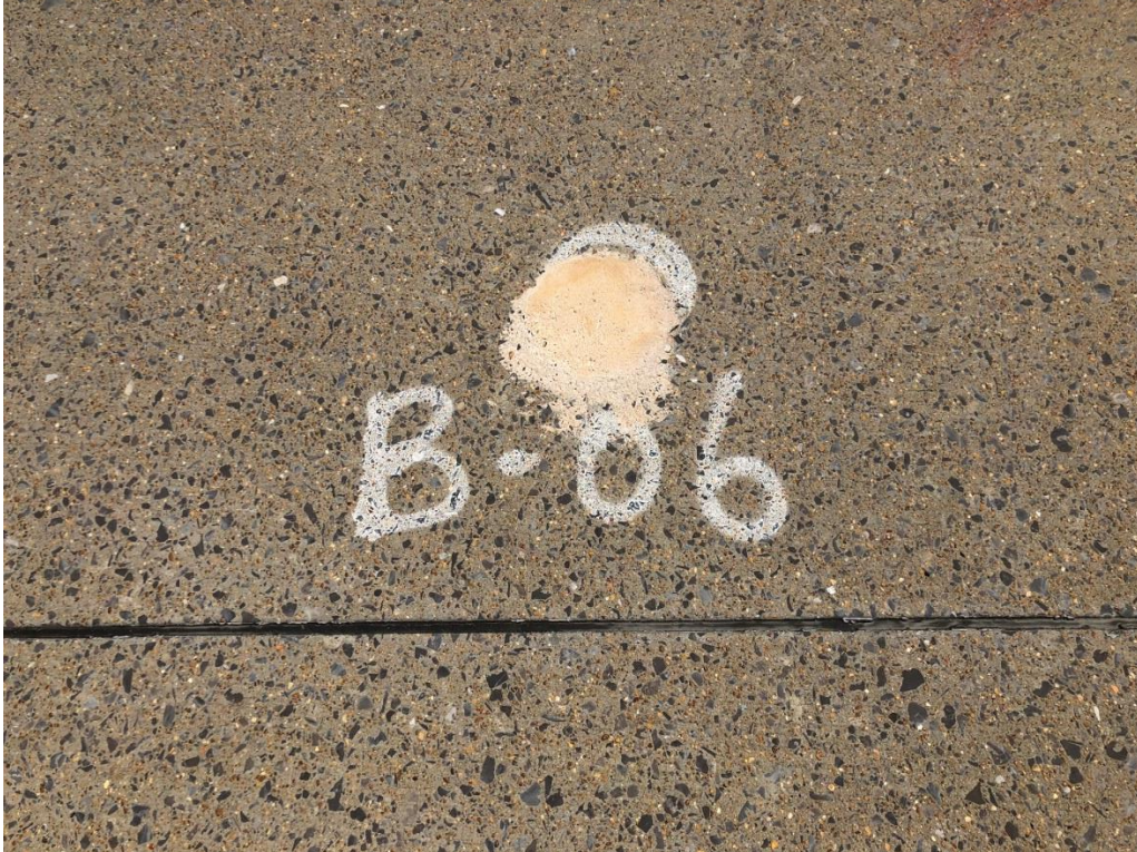
Geotechnical Boring # 6
