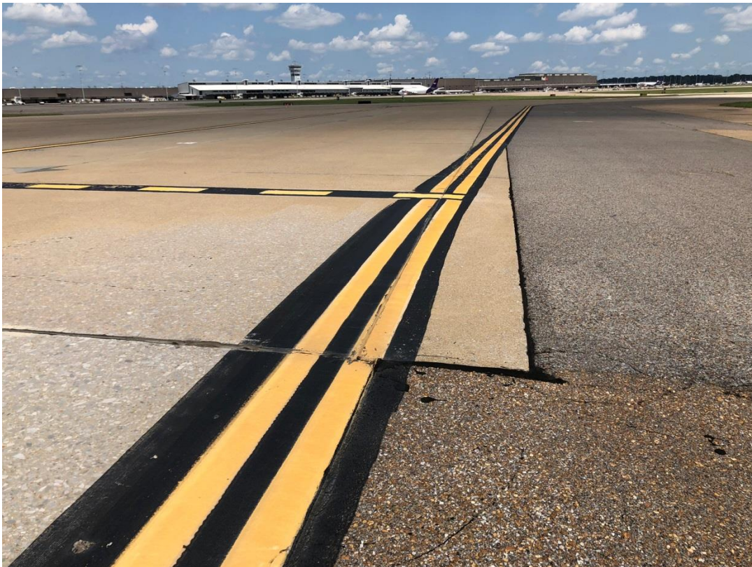
Delpatch repairs along Taxiway Bravo
