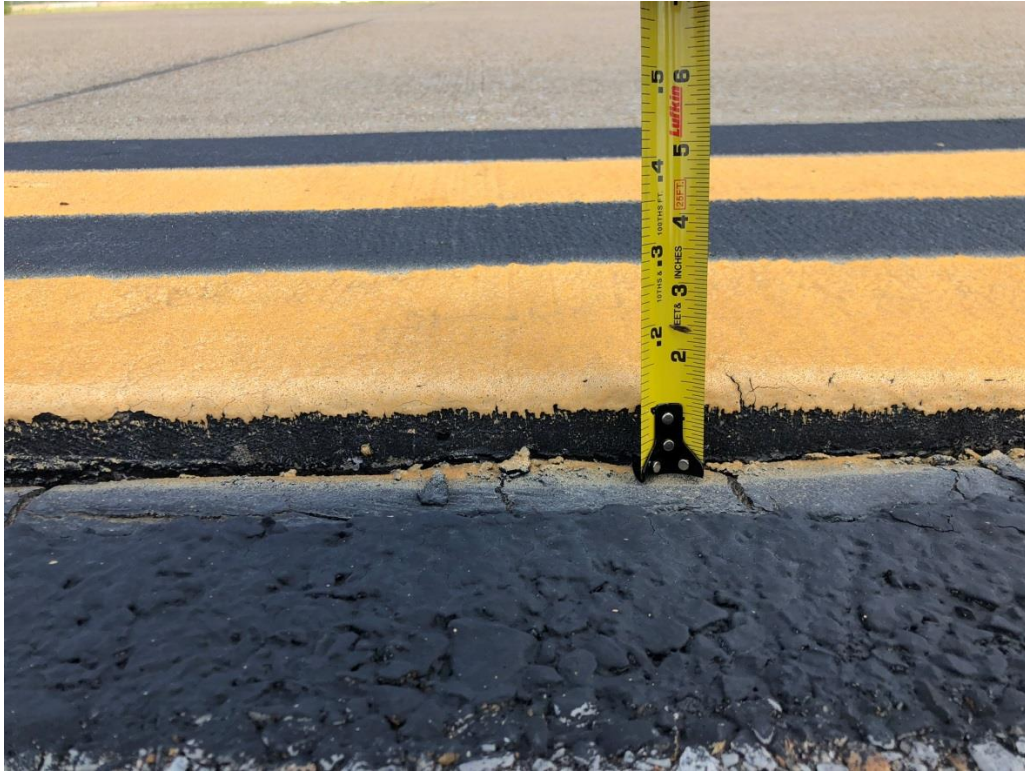
Inch and a half drop off at existing PCC pavement/asphalt shoulder interface
