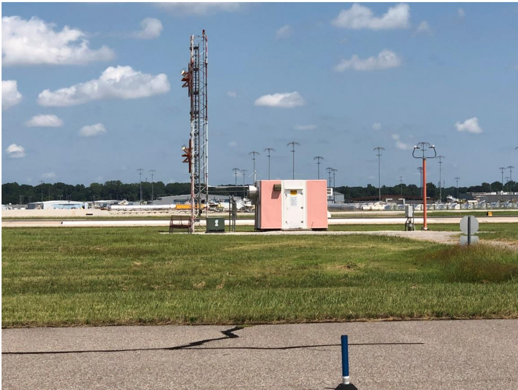
Glide Slope Antenna for Runway 9
