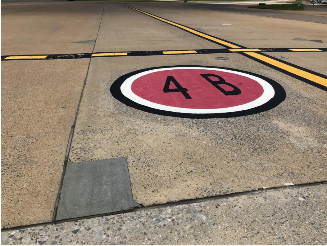
Delpatch repairs along Taxiway Bravo
