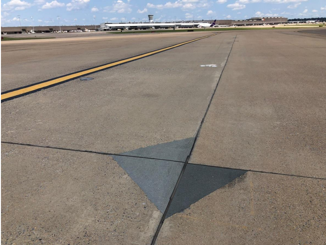
Taxiway Bravo Delpatch Repairs with joint sealant
