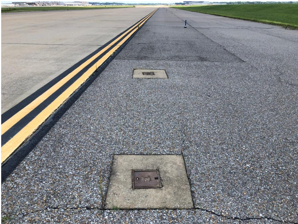
Typical underdrain cleanout
