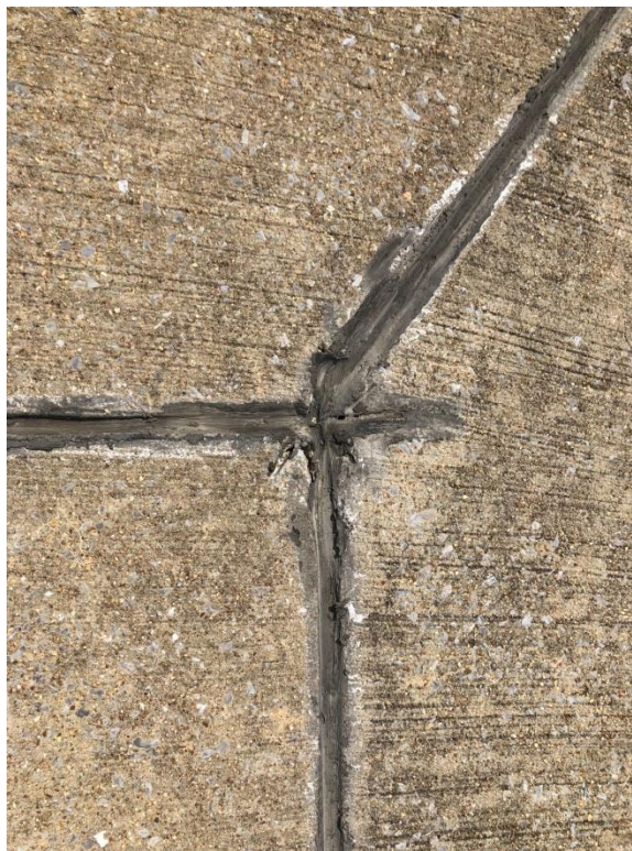
Typical concrete joint and sealant
