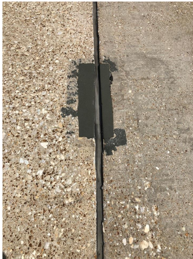
Typical Delpatch Elastomeric Concrete repair (typical)
