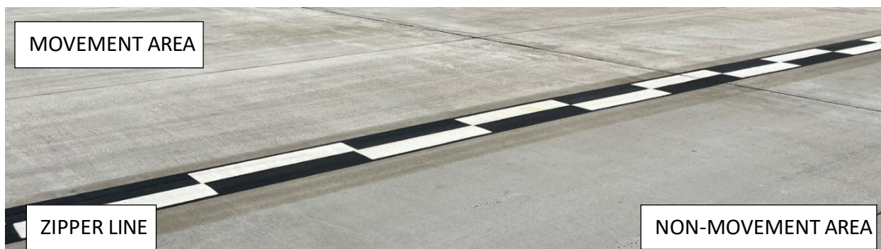
Figure 5 – Dashed Taxiway Edge Markings and Black/White Zipper Marking
