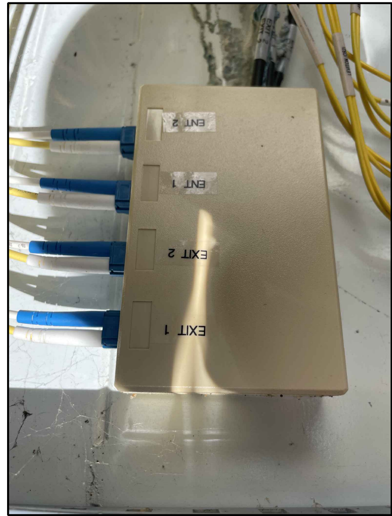
EXISTING FIBER OPTIC PATCH PANEL
