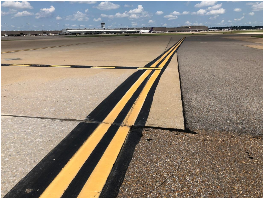
Delpatch repairs along Taxiway Bravo
