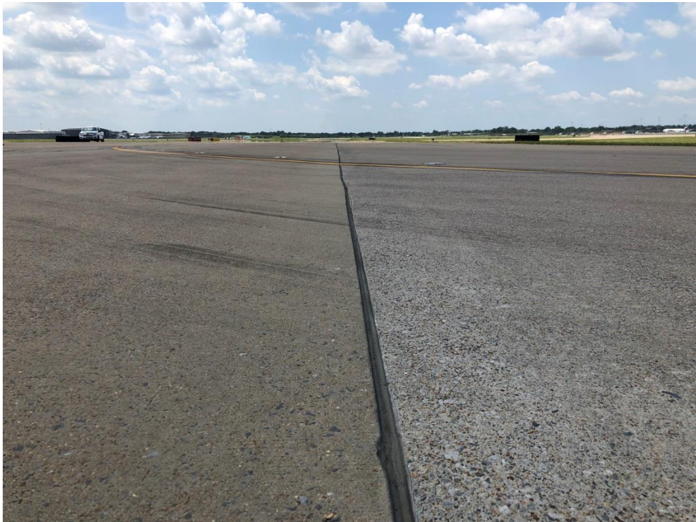
Proposed tie-in joint @ Bravo looking west. Right half remains
