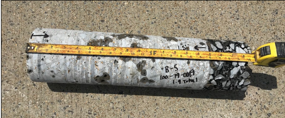
Photo 13: Concrete Core Location B-5
