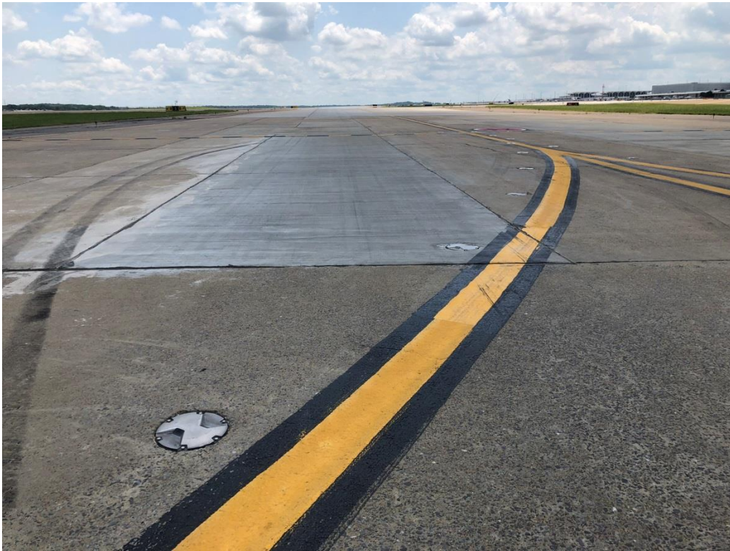
PCC Panel Replacement on Taxiway Sierra looking South
