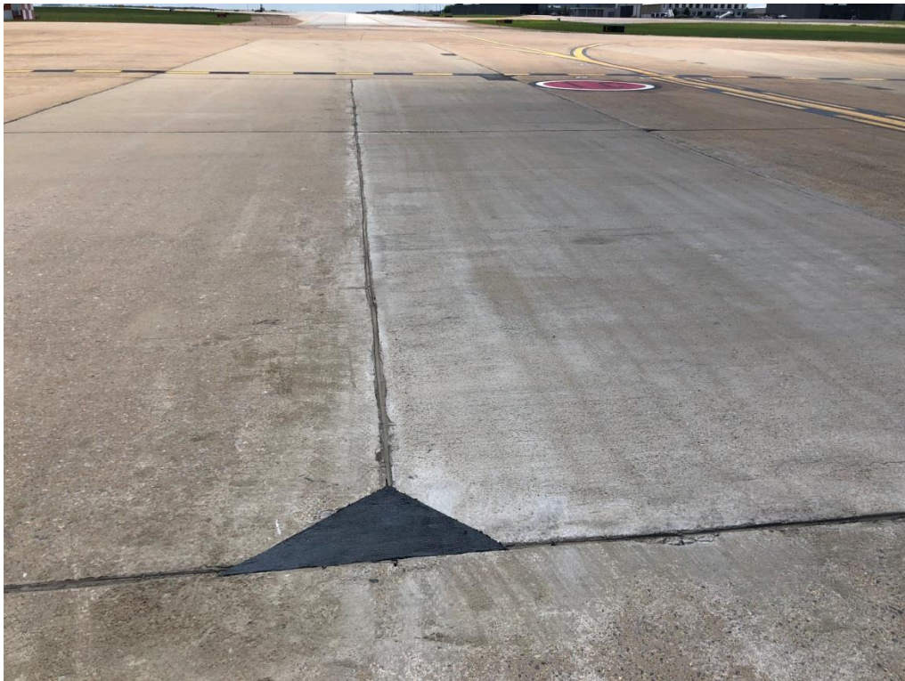
Corner Repair along Taxiway Charlie
