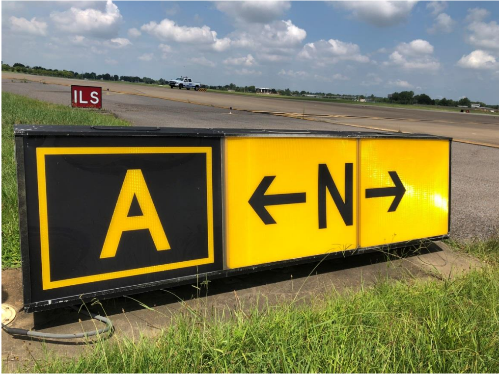
Taxiway Guidance Sign
