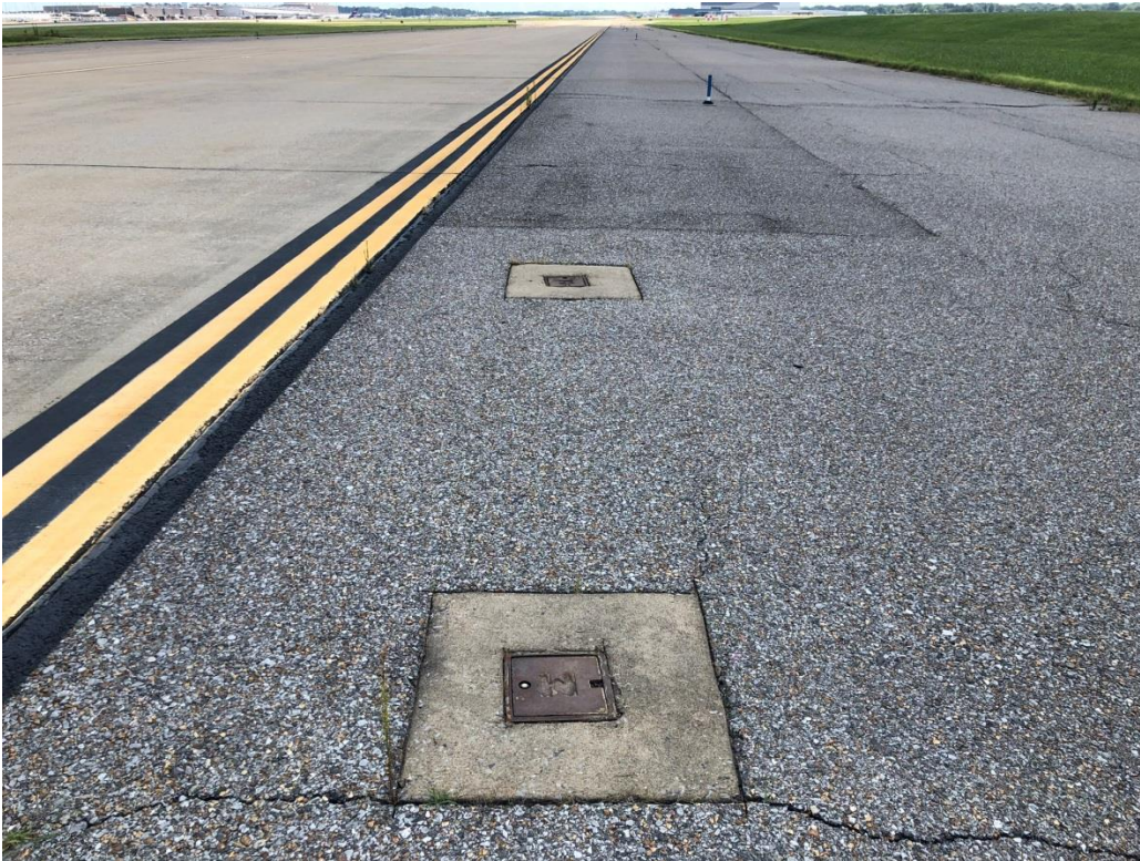
Typical underdrain cleanout
