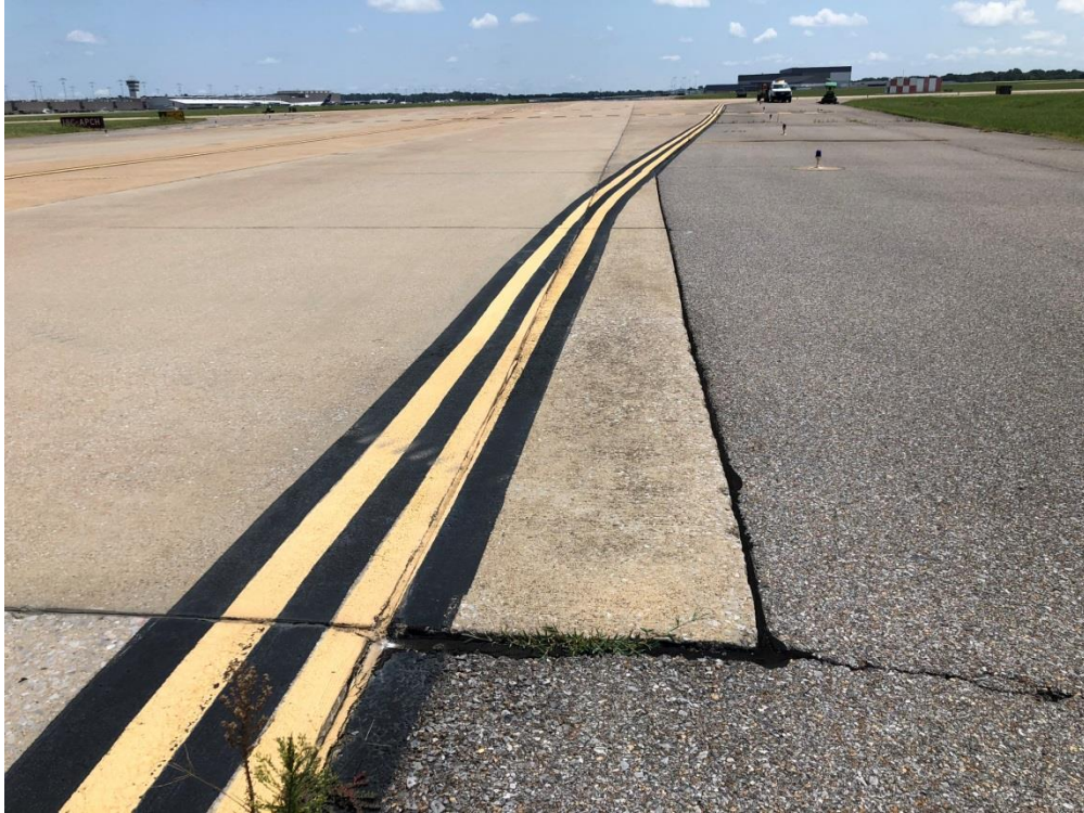
Beginning of edge fillet for Taxiway Charlie
