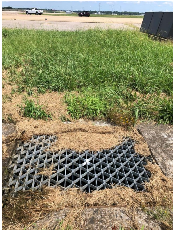
Existing Inlet Grate near Taxiway Alpha/November intersection
