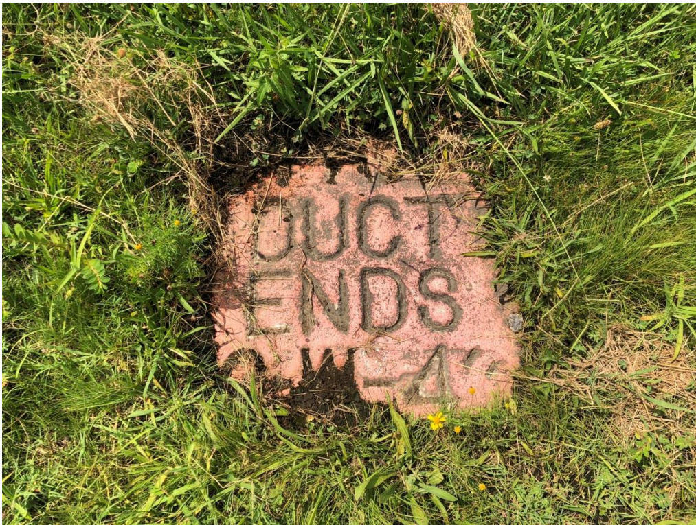
Duct end marker along Taxiway Alpha @ November intersection
