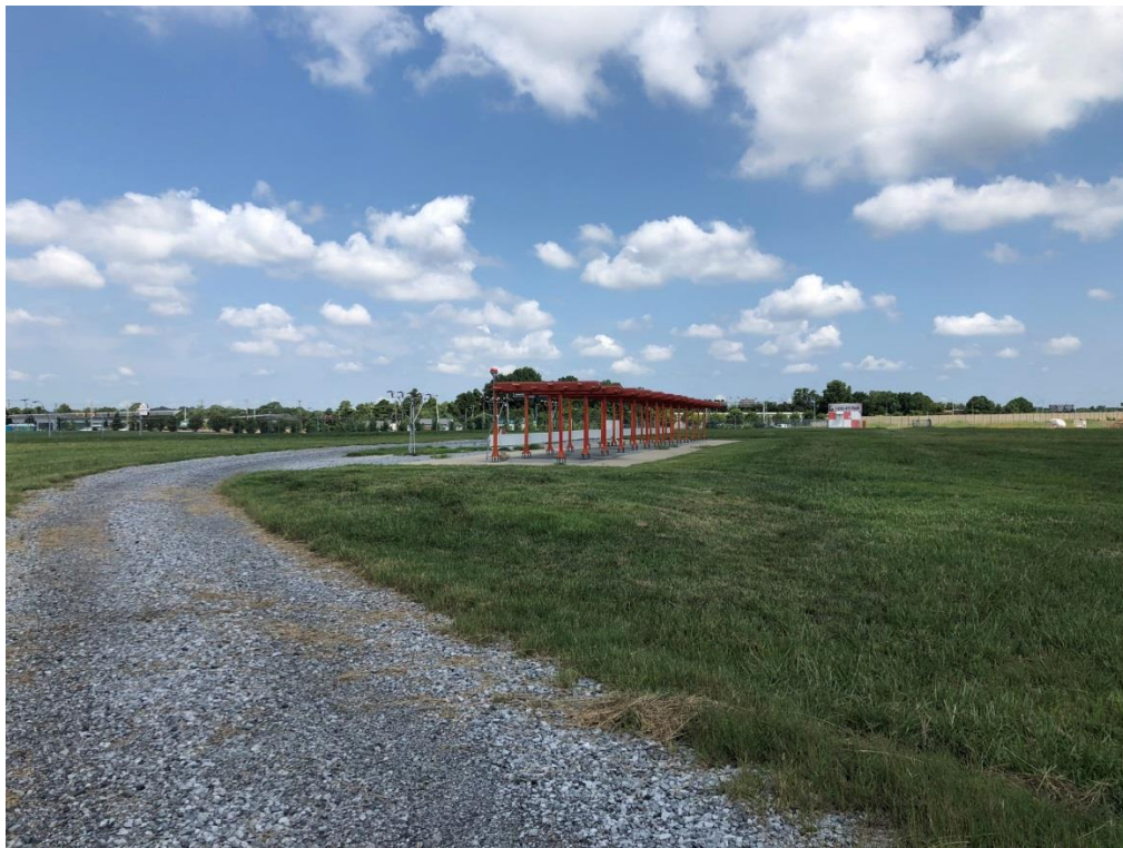
Runway 9 Localizer Antenna and access drive
