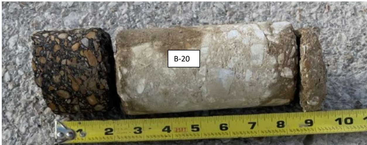
Photo 2: Concrete Core Location B-20
