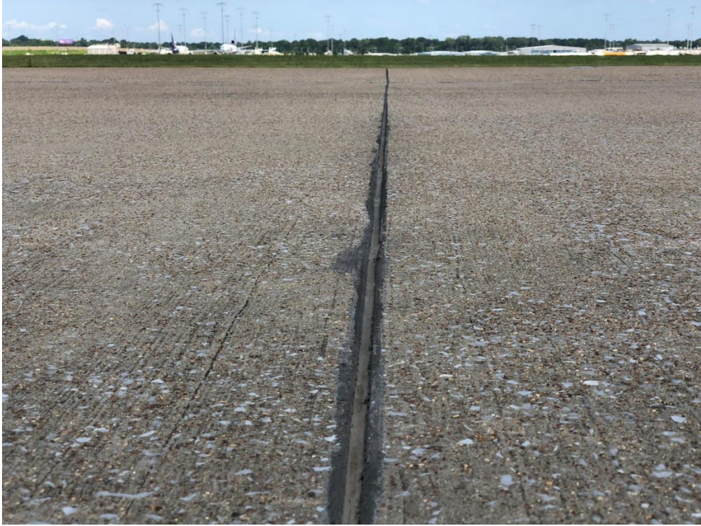
Typical PCC joint
