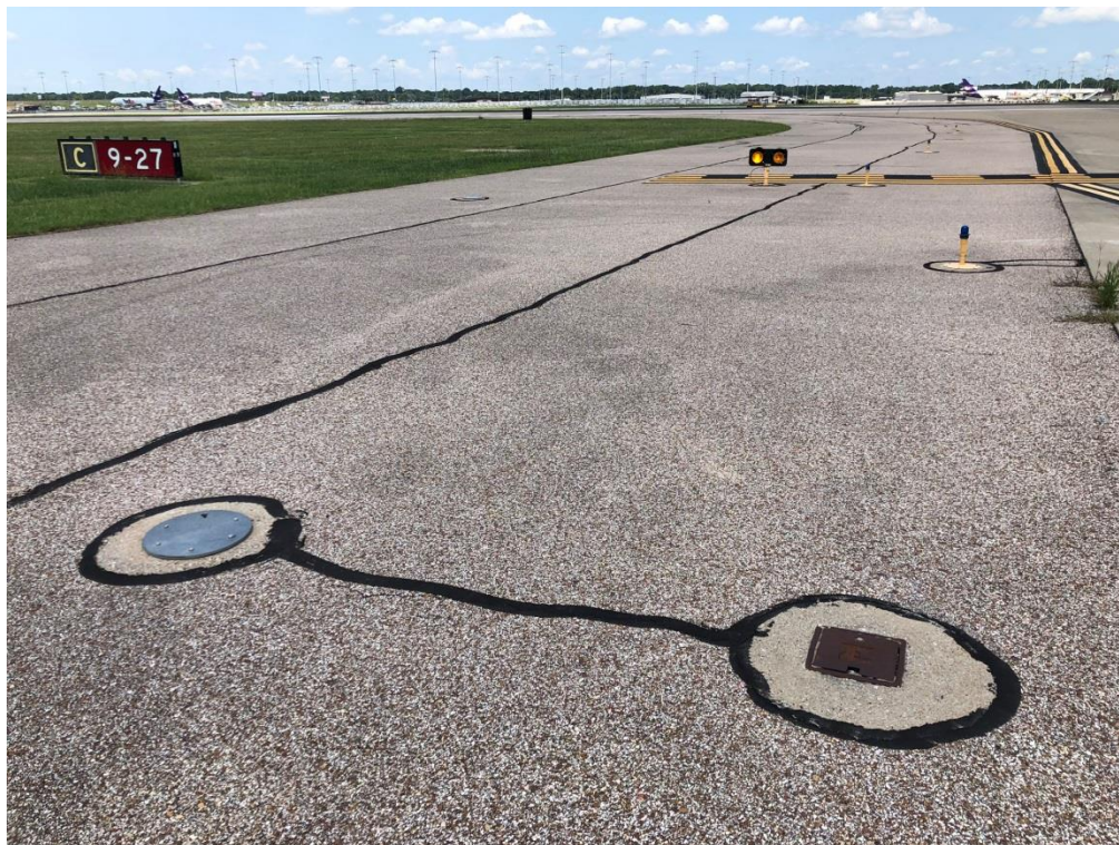
Along Taxiway Charlie looking north towards 9-27 Hold
