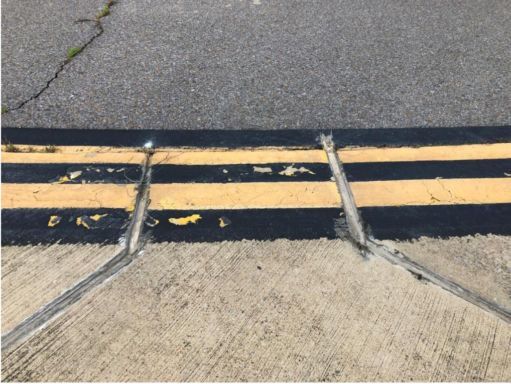
Typical slab joint transition
