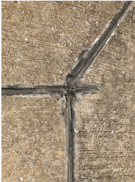
Typical concrete joint and sealant
