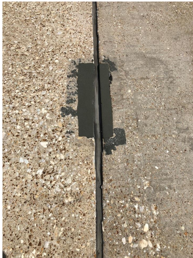
Typical Delpatch Elastomeric Concrete repair (typical)
