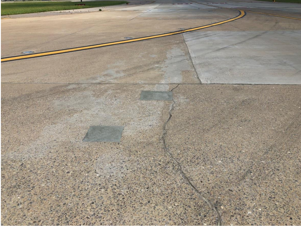
Repairs @ mid-intersection of Taxiway Sierra and Taxiway Alpha
