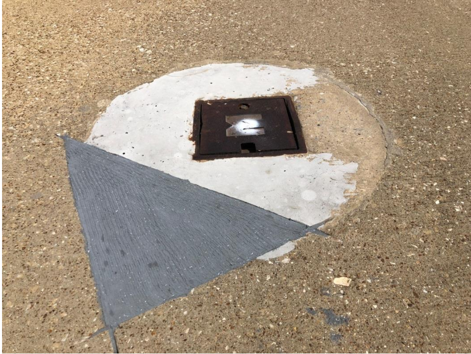
Delpatch surrounding existing cleanout
