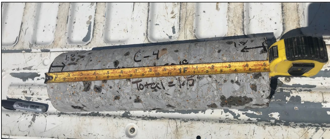
Photo 3: Concrete Core Location C-4
