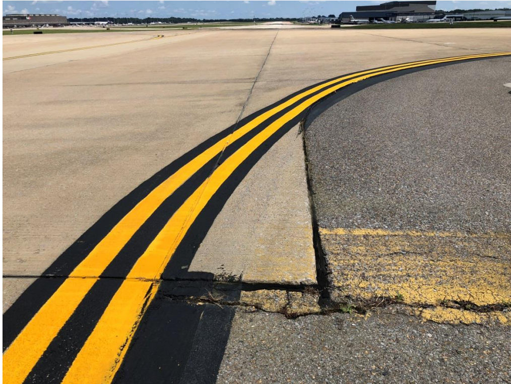
Fillet widening along Taxiway Alpha for southern radius
