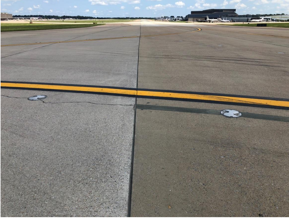
Proposed tie-in joint at Taxiway Bravo Intersection (left half remains)
