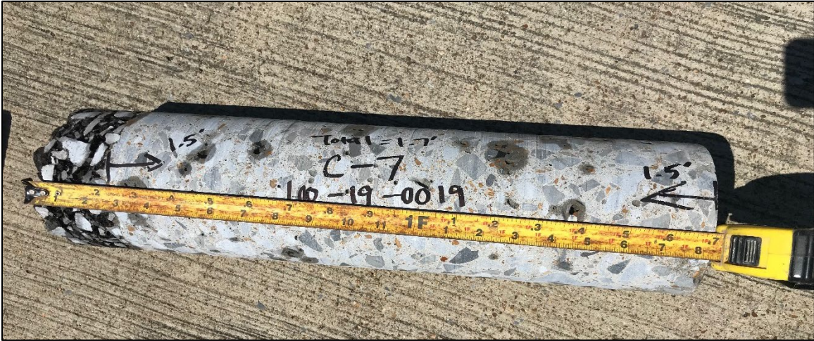
Photo 4: Concrete Core Location C-7
