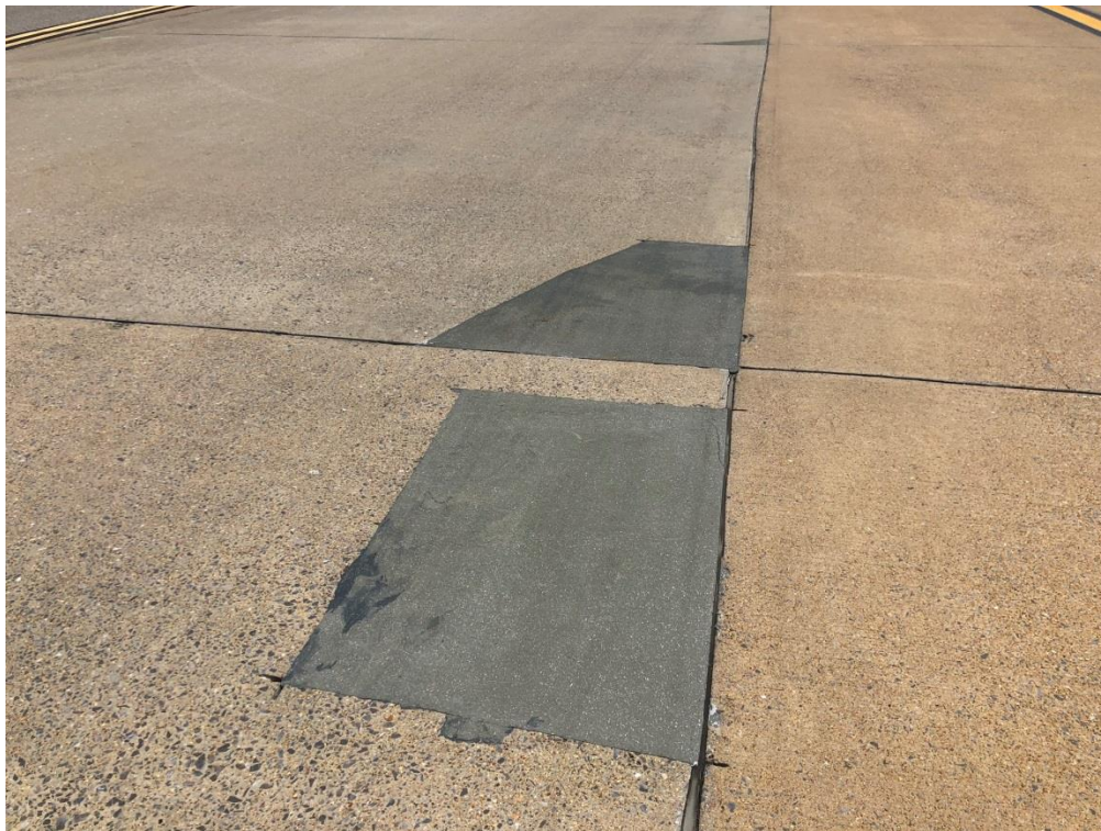
“Delpatch” Repairs along Taxiway Alpha near Taxiway Charlie
