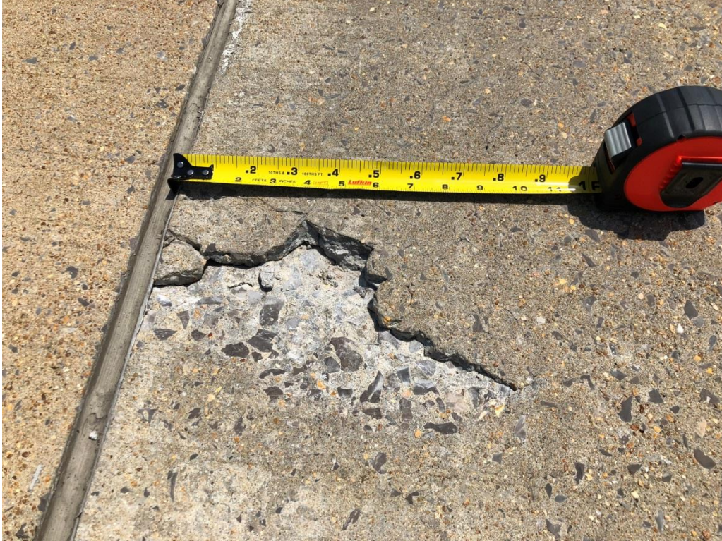
Joint Spalling
