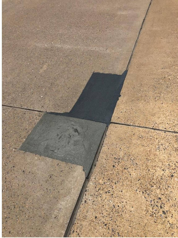
Delpatch corner break/spall repair
