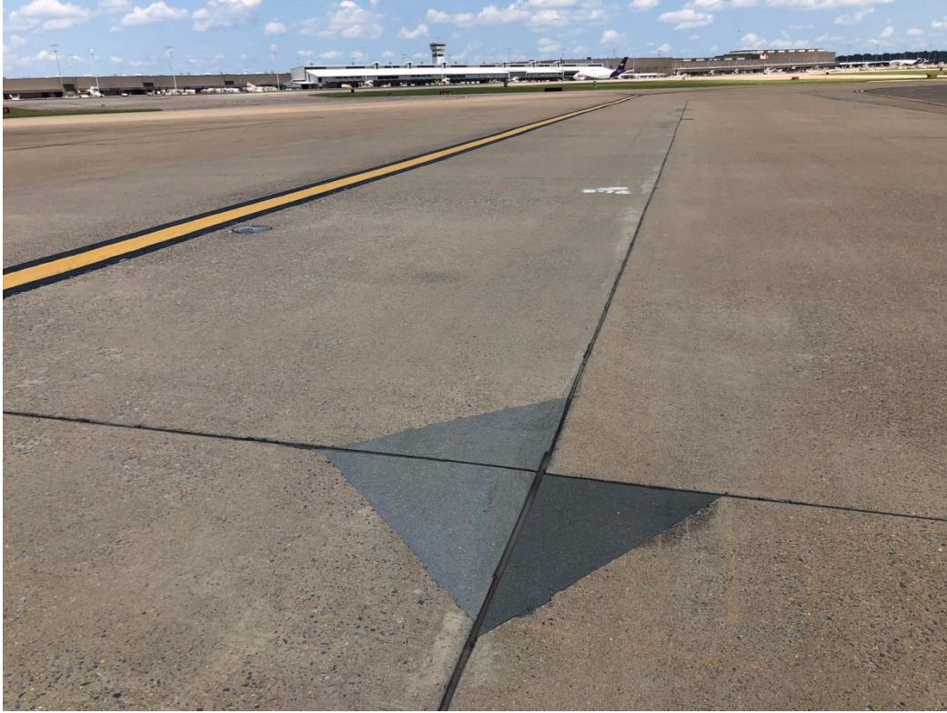
Taxiway Bravo Delpatch Repairs with joint sealant
