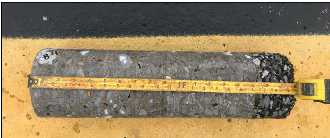
Photo 12: Concrete Core Location B-4
