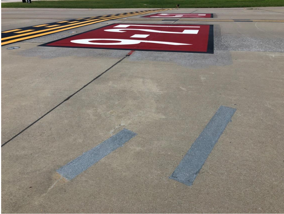
Taxiway Charlie repairs near 9-27 Hold
