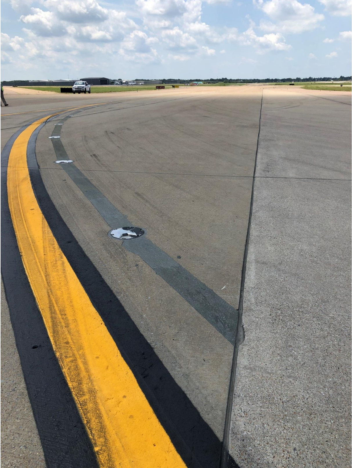
Taxiway Bravo @ Proposed tie-in joint (Right half remains)
