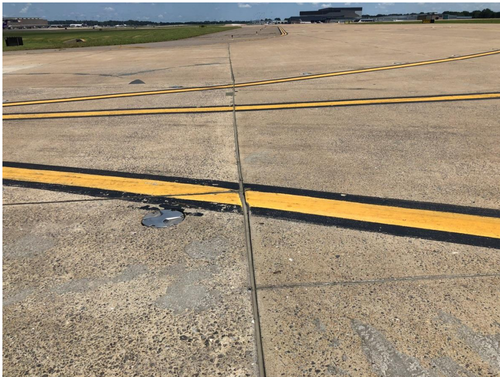
Thickened-edge expansion joint along Taxiway Alpha
