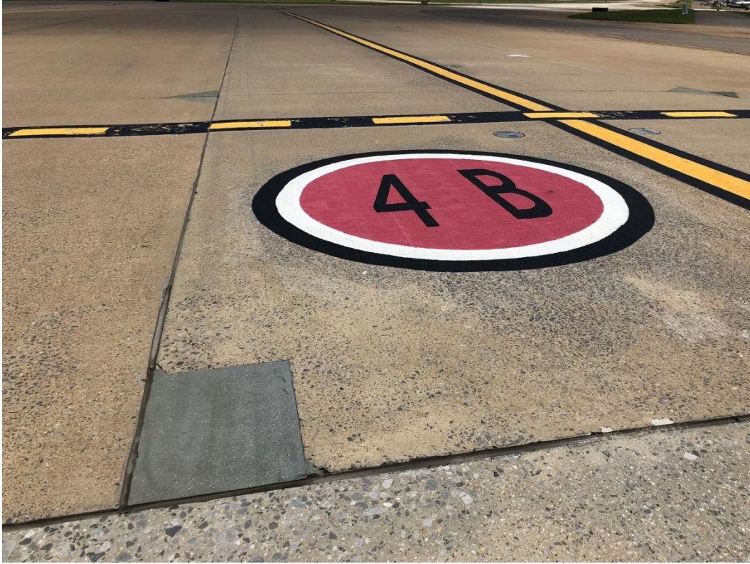
Delpatch repairs along Taxiway Bravo
