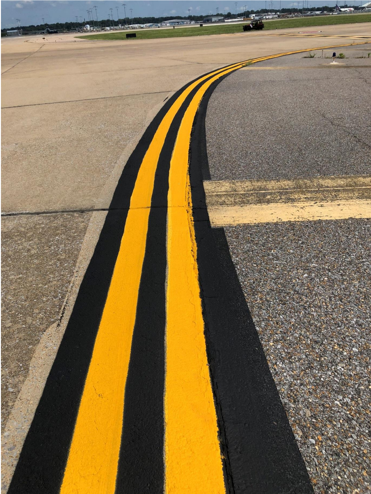
Existing taxiway edge striping and shoulder striping at Alpha/November intersection
