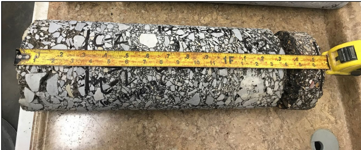
Photo 2: Concrete Core Location C-2
