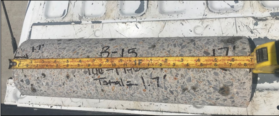
Photo 22: Concrete Core Location B-15
