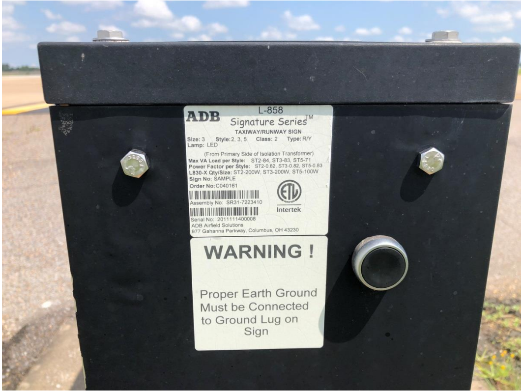
Existing Taxiway Signage (Typical)
