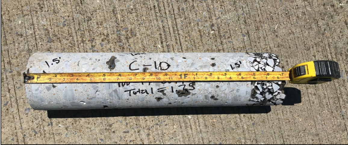
Photo 7: Concrete Core Location C-10
