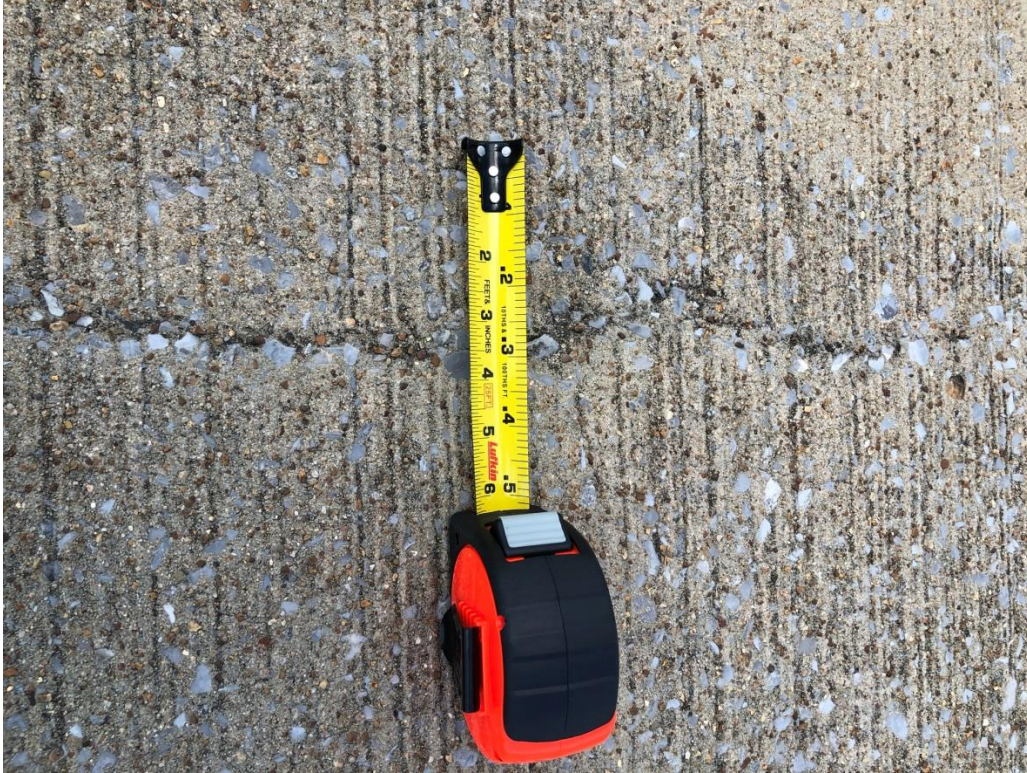
PCC Cracking
