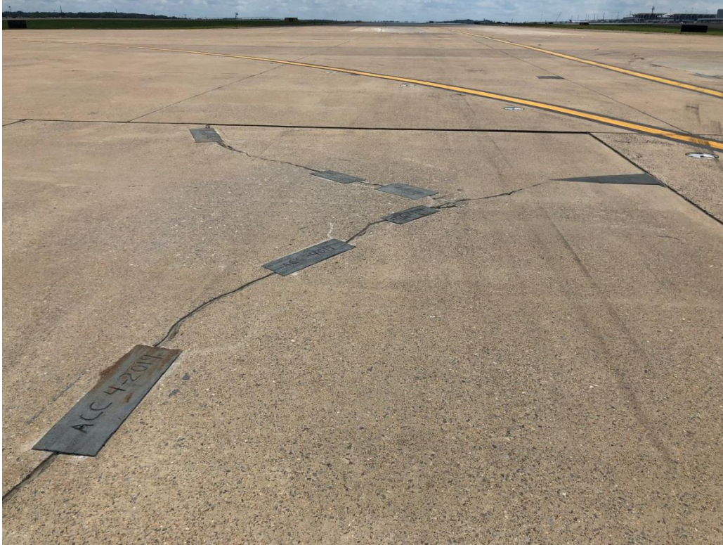
Crack Repair along Sierra looking South
