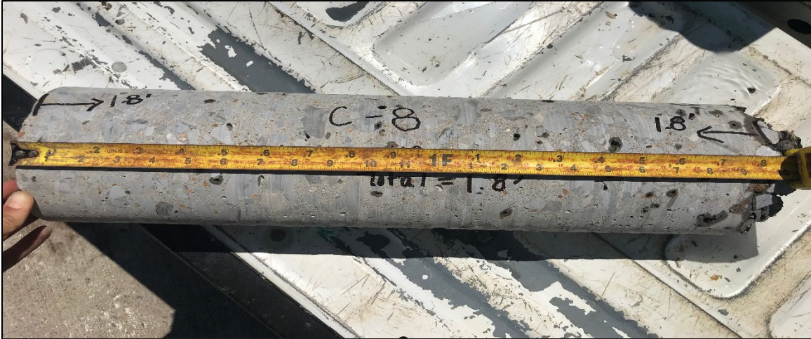
Photo 5: Concrete Core Location C-8
