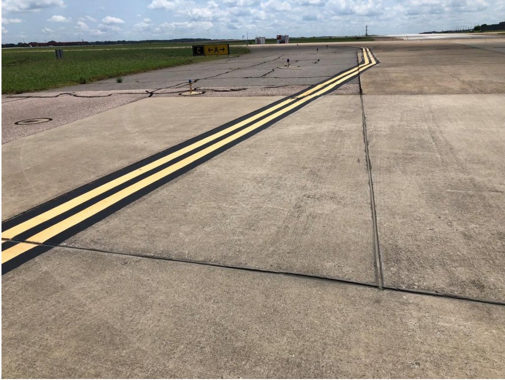
East fillet widening of Taxiway Charlie looking South towards Taxiway Alpha
