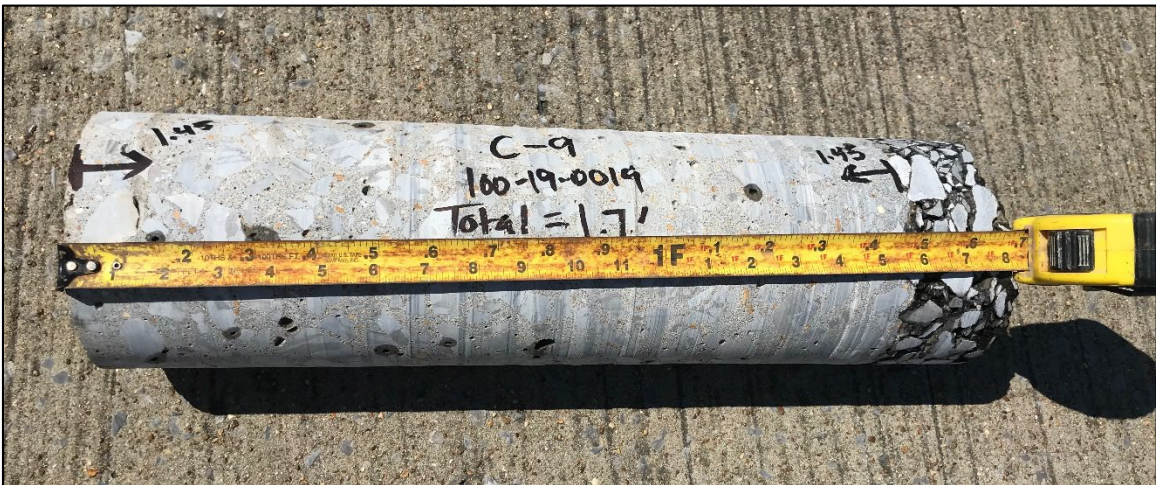
Photo 6: Concrete Core Location C-9
