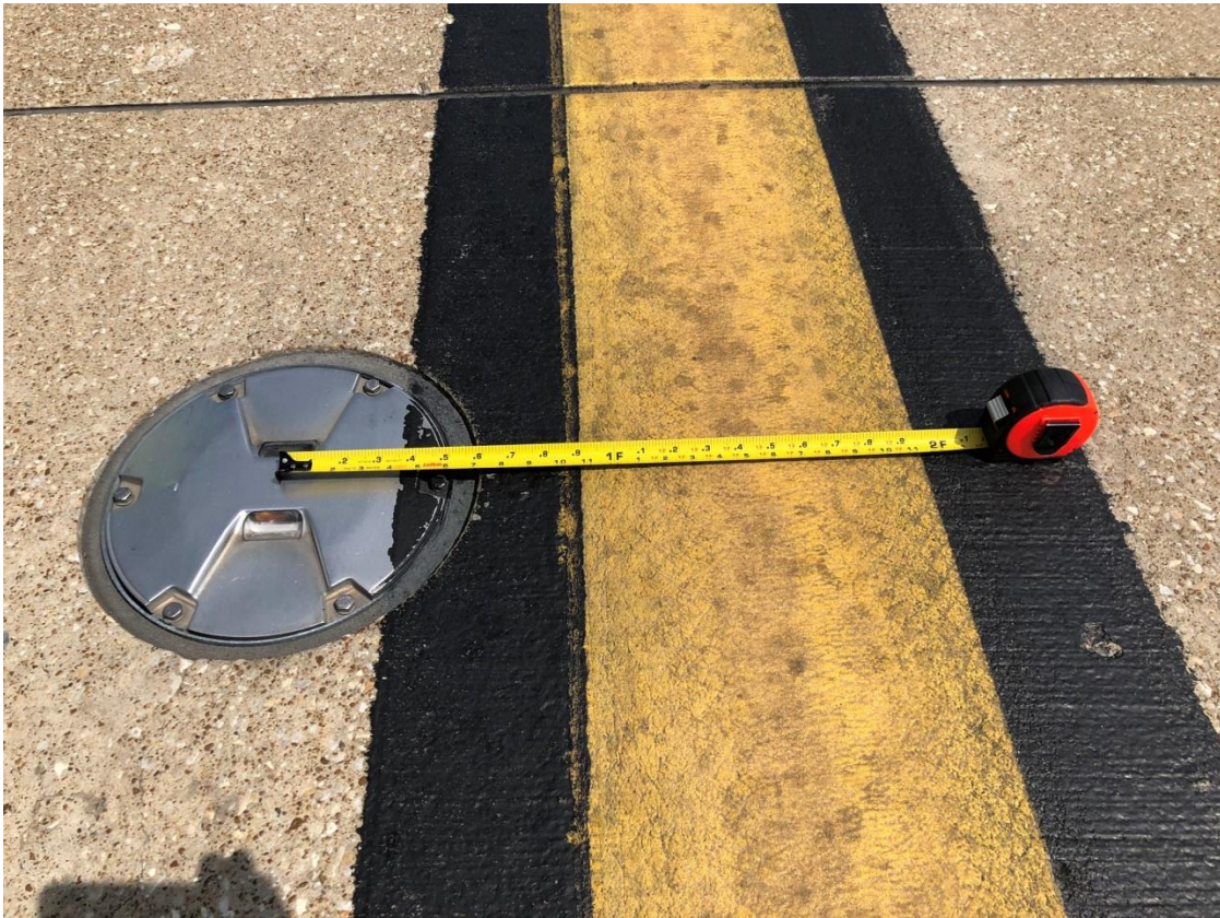
Existing centerline light can approximately 1.5' off centerline stripe
