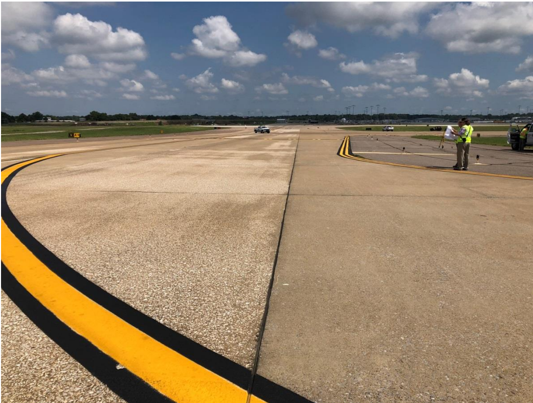
Looking north up Taxiway November at tie-in joint
